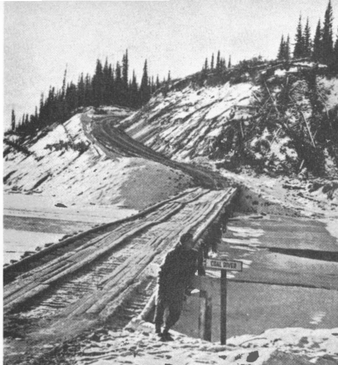
FIGURE 61 Typical temporary bridge on pioneer trail of the Alaska Highway.
