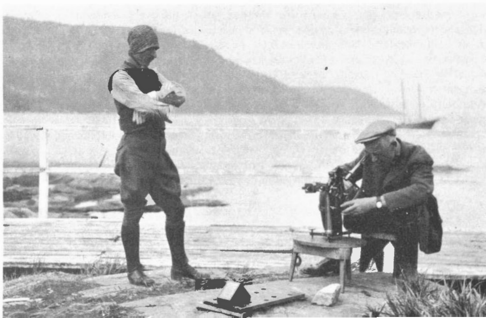
FIGURE 67. Captain Frederick Anderson (seated) using sextant and artificial horizon at Rigolet, Hamilton Inlet, 1921. G.-A. Bachand, at left, was drowned 10 years later in Netagamu River.
