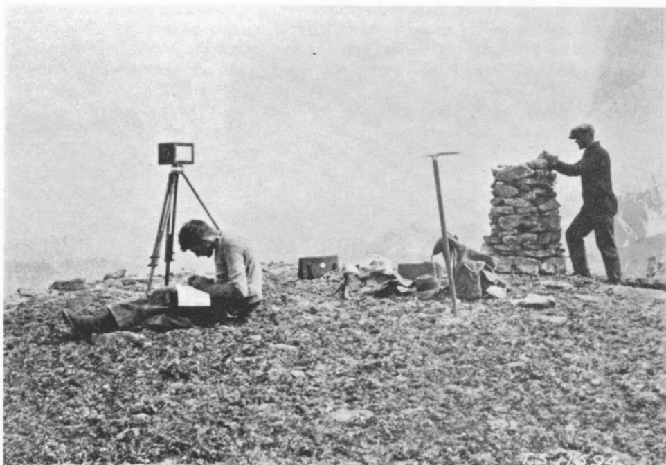
FIGURE 4. Surveyors marking site of a photo-topographical mapping station with stone cairn in mountain country, 1929.
