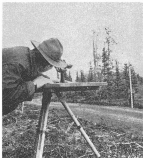
FIGURE 66 Levelling operations along the Alaska Highway, Geodetic Survey of Canada.
