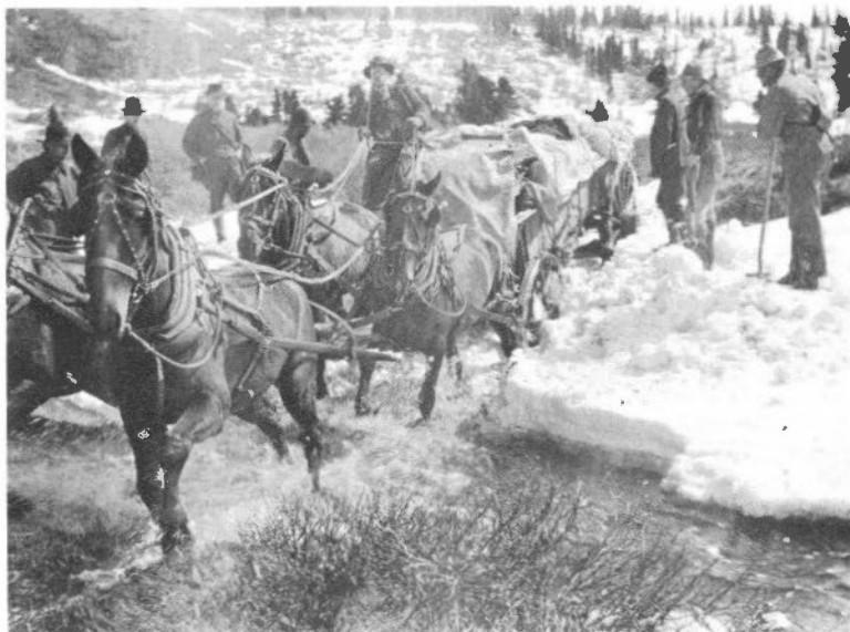
FIGURE 80. Surveyors en route to boundary line, west of Whitehorse, Y.T., 1909.
