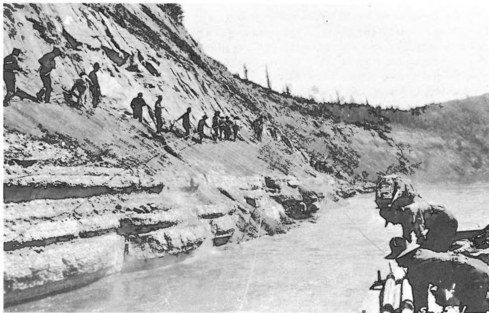
FIGURE 54. 'Lining' survey barges upstream in swift water, 1900.
