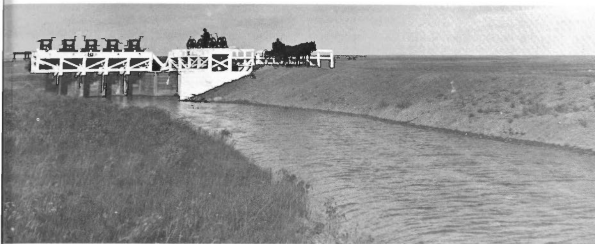
FIGURE 45. Head gates and reservoir on C.P.R. irrigation system in Southern Alberta.
