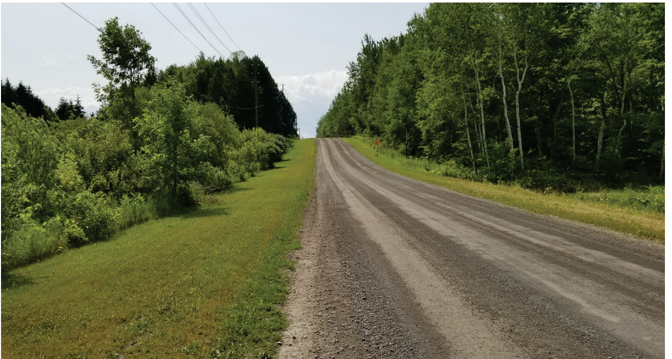
Fig. 17 Photo of possible toe of landslide debris deposition zone (taken from WT01 on July 10, 2018, facing south. See Fig. 14 for location. Note road sloping up from where the photo is taken)
