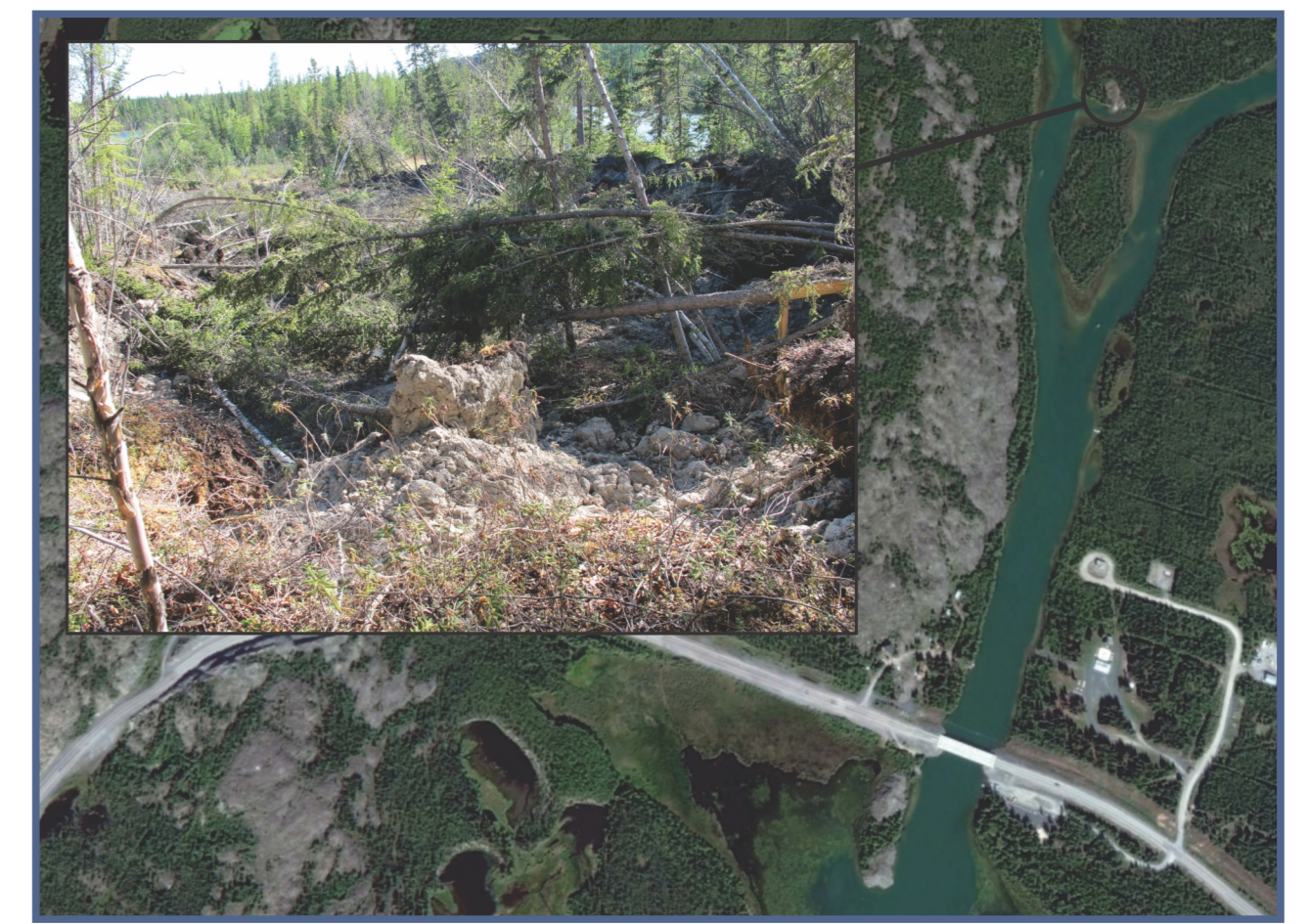
Figure 6. Retrogressive thaw slump on the Yellowknife River, north of NWT Highway 4, east of Yellowknife, NT. Inset shows the debris flow below the headwall.
