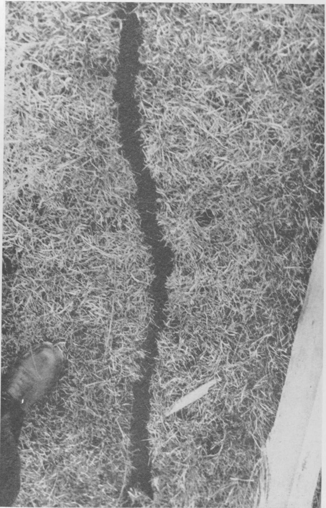
FIG. 17.—Slump crack in ground near Rivière Ouelle church
