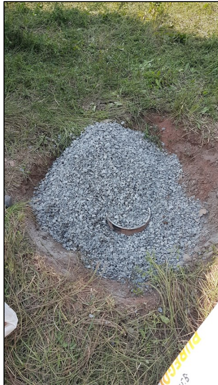
Figure B.12 - Observation well PO-05 after its decommissioning (step 5) (August 25, 2018)
