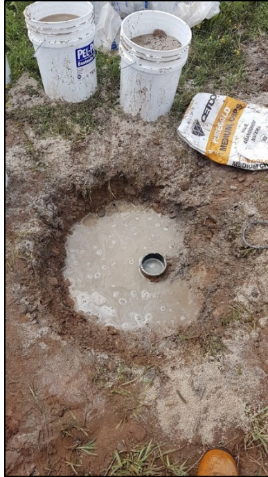
Figure B.27 - Observation well PO-13 during its decommissioning (step 4) (August 26, 2018)
