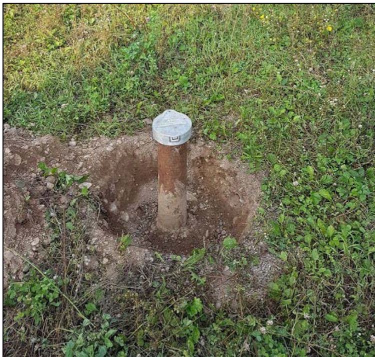
Figure B.22 - Observation well PO-09 during its decommissioning (step 1) (August 25, 2018)
