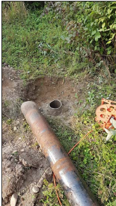
Figure B.14 - Observation well PO-06 after step 2 (casing cutoff) (August 25, 2018)
