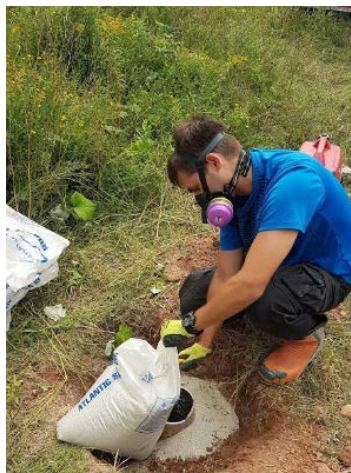
Figure 6 - Pouring of sand in the well
