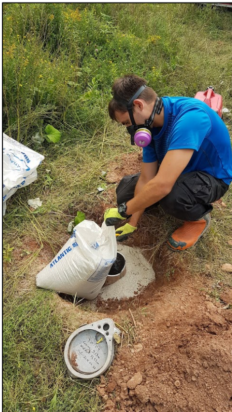
Figure B.9 - Observation well PO-04 during its decommissioning (step 3) (August 24, 2018)
