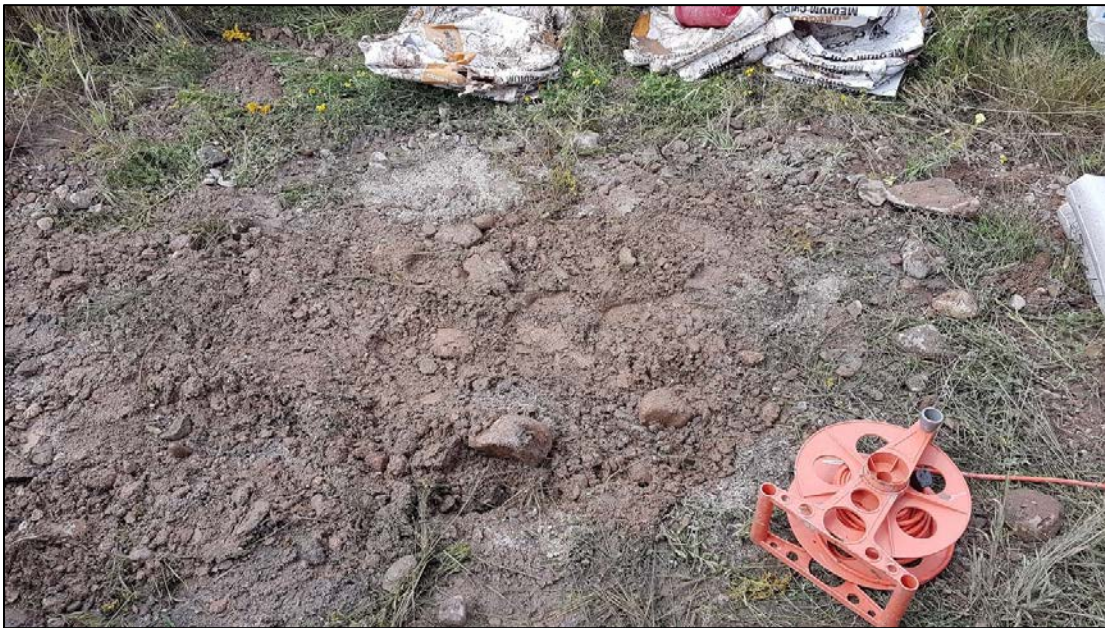
Figure B.8 - Observation well PO-02 after its decommissioning (August 26, 2018)
