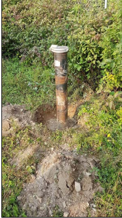
Figure B.13 - Observation well PO-06 before its decommissioning (August 25, 2018)
