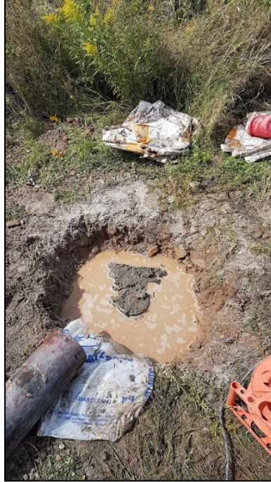
Figure B.7 - Observation well PO-02 completely filled (end of step 4) (August 26, 2018)
