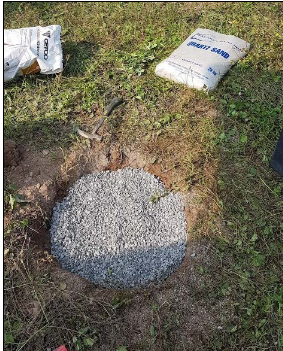
Figure B.24 - Observation well PO-09 in the decommissioning final stage (step 5) (August 25, 2018)
