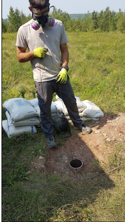
Figure B.11 - Observation well PO-05 during its decommissioning (step 3) (August 25, 2018)
