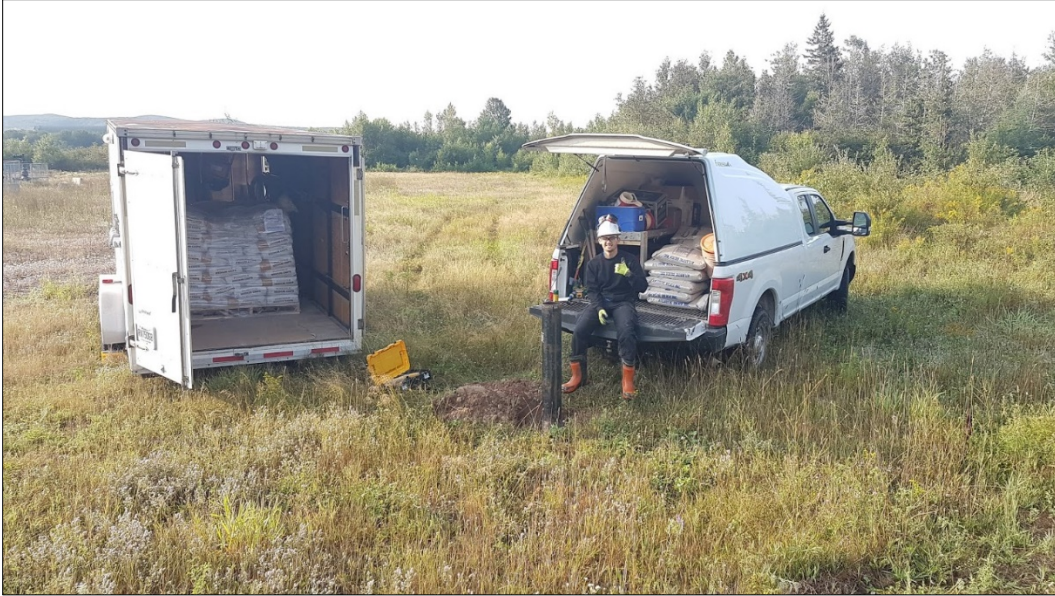
Figure B.1 - Observation well PO-01 before its decommissioning (August 24, 2018)
