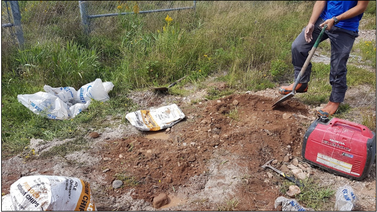
Figure B.29 - Observation well PO-13 after its decommissioning (August 26, 2018)
