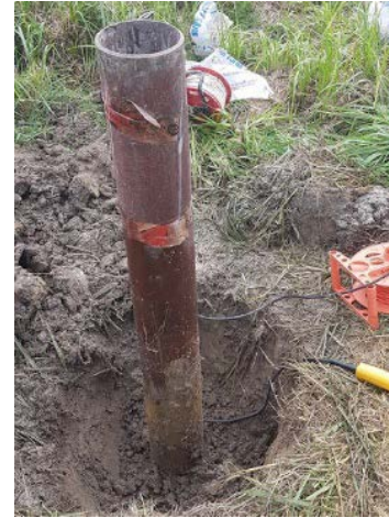
Figure 4 - Hole dug around the well
