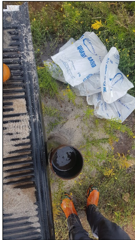
Figure B.6 - Observation well PO-02 during decommissioning (step 3) (August 26, 2018)
