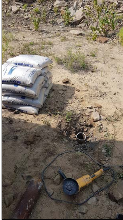
Figure B.19 - Observation well PO-08 during its decommissioning (step 2) (August 25, 2018)
