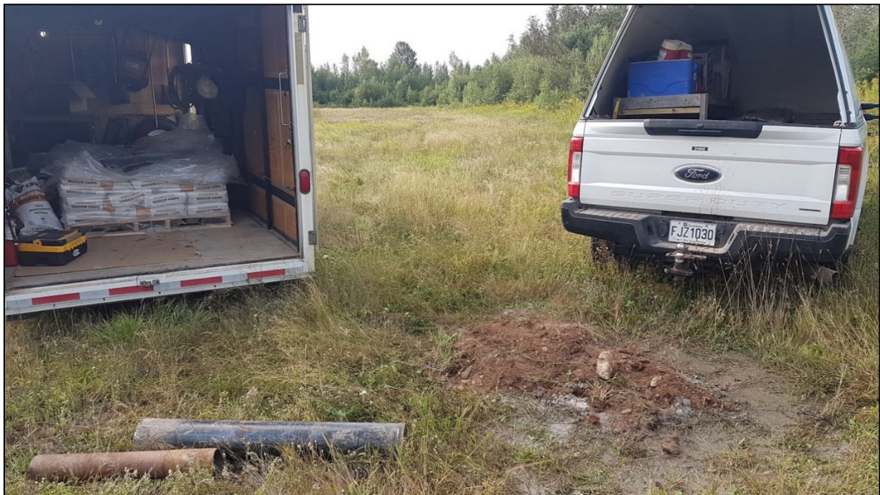
Figure B.4 - Observation well PO-01, after its decommissioning (August 24, 2018)
