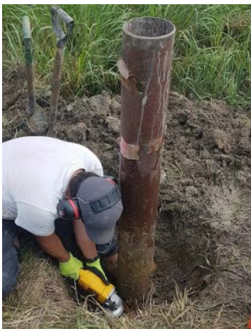
Figure 5 - Cutting of the casing
