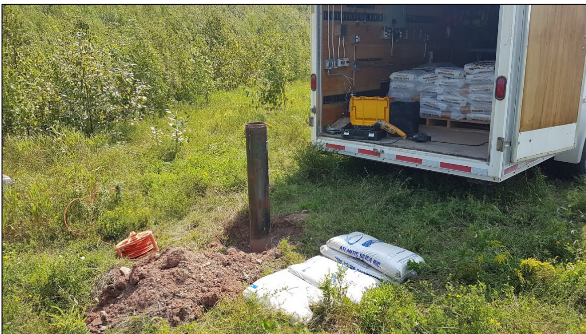
Figure B.10 - Observation well PO-05 before its decommissioning (August 25, 2018)
