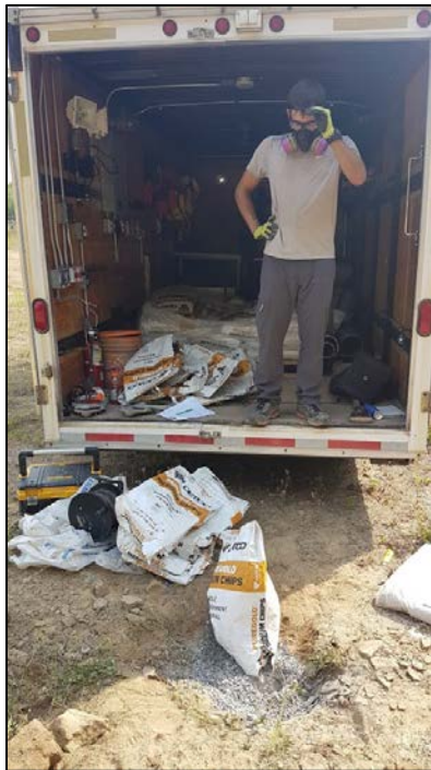
Figure B.20 - Observation well PO-08 during its decommissioning (step 5) (August 25, 2018)
