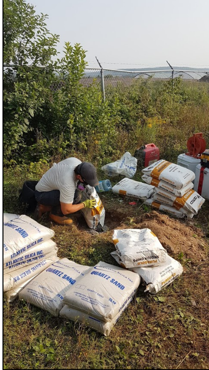
Figure B.23 - Observation well PO-09 during its decommissioning (step 4) (August 25, 2018)
