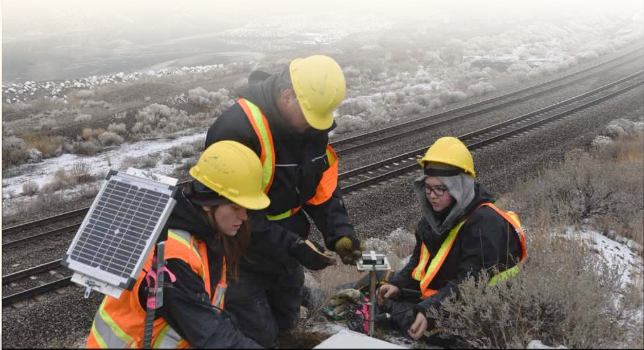
The GSC conducts geohazard studies to reduce risks to people and infrastructure, here installing equipment to monitor landslide activity above a critical railway corridor in central BC.
