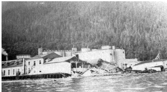
Figure S5-7 Damage at the Woodfibre mill attributed to tsunami generated by submarine mass movement (source: Squamish Museum archives).
