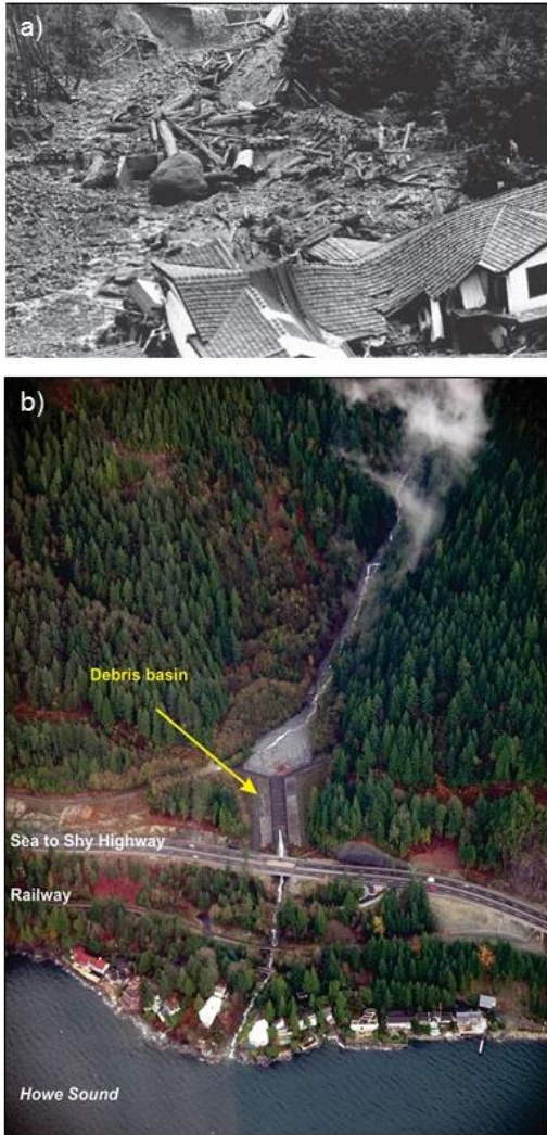
Figure S6-3 a) Debris torrent damage at Lions Bay from the 1981 event (source: Turner et al. 2010); b) debris basin at Charles Creek (source: O. Hung).
