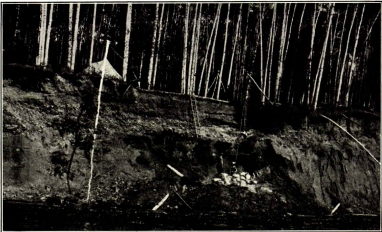
Preliminary excavation of outcrop of bituminous sand on Horse creek.
