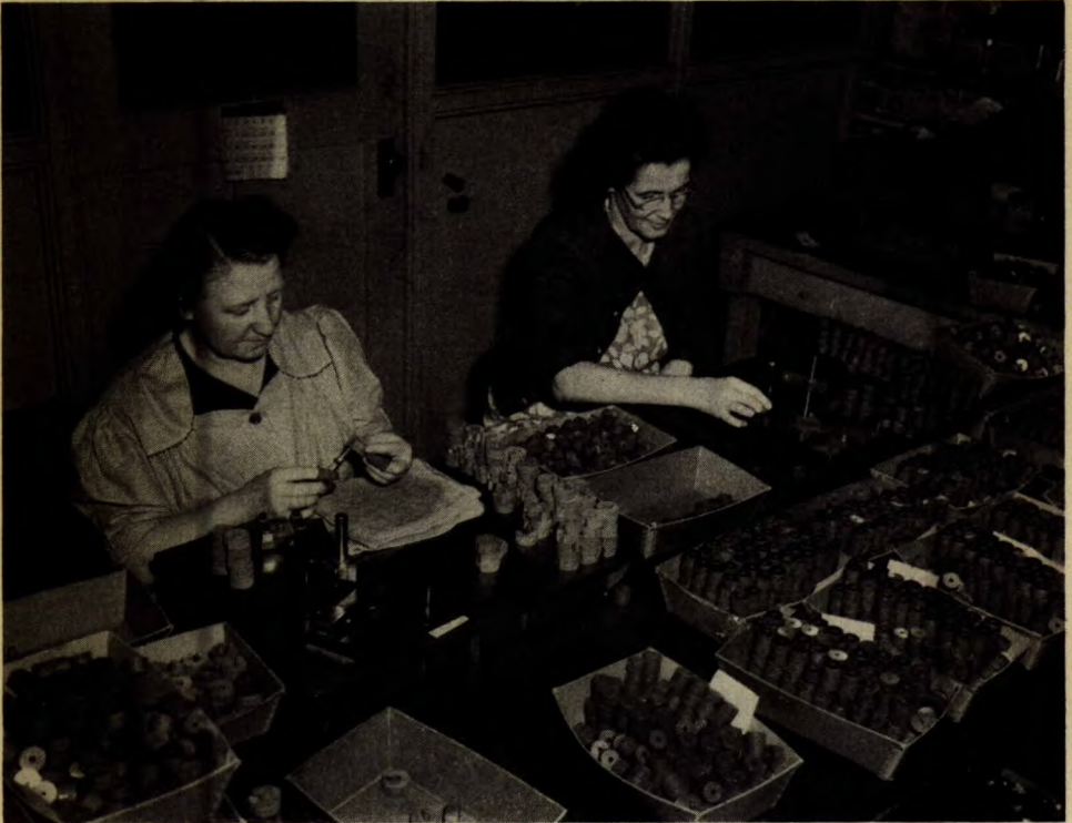
FIGURE XXII. Inspection of precision-cast Alnico magnets.
