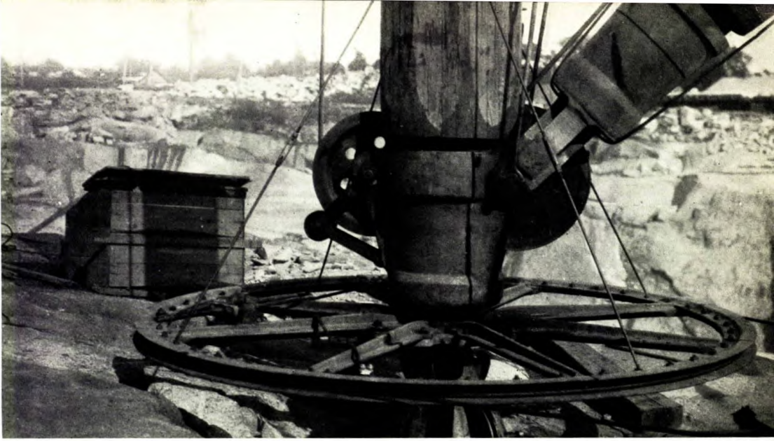
Figure 25 | Details at base of large derrick, Brodie's Limited quarry, Graniteville, Quebec.
