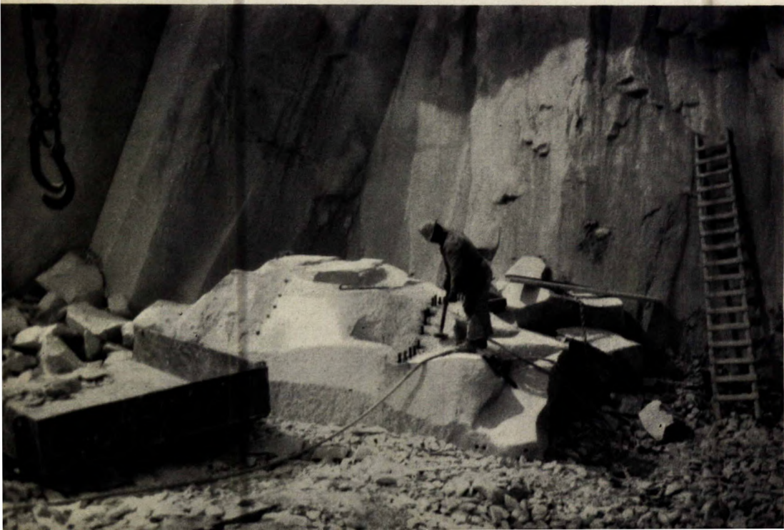
Figure 41 | Subdividing by 'plug and feather', Haddington Island, B.C.
