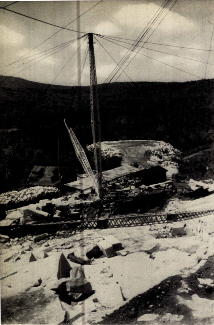
Figure 32 | Derricks at Deschambault Quarry Co. poration quarry, 5 miles east of St. Gérard, Que.
