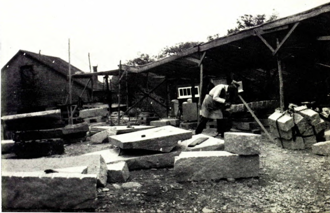
Figure 34 | Hand dressing granite blocks. St. Samuel Granite quarry, St. Samuel-St. Sébastien District, Que.
