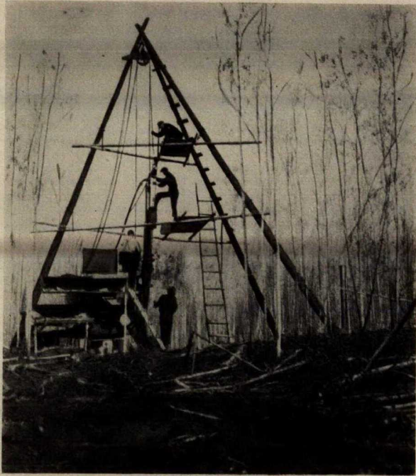
A. Drilling in the Steepbank area, Alberta.
