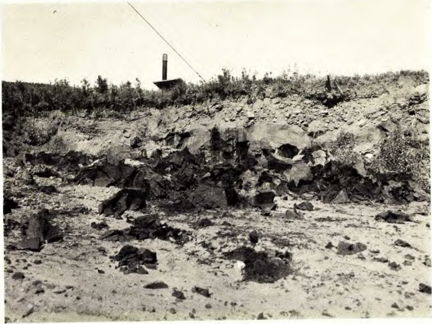
A. Blasting bituminous sand at plant of Abasand Oils, Limited, McMurray, Alberta.
