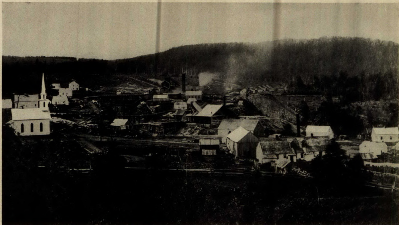
Albert Mines, New Brunswick, at time of mining albertite vein.
