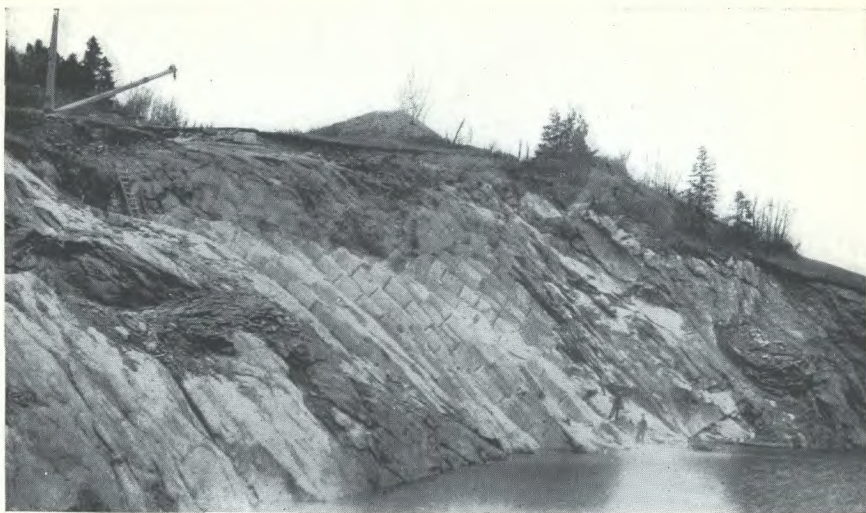
A. View of soapstone quarrying operation along north side of old open pit of Kitchener asbestos mine, range V, lot 2, Thetford Township, Megantic County, Que. Illustrates the occurrence of a band of soapstone as a marginal deposit bordering a body of asbestos-bearing serpentine.
