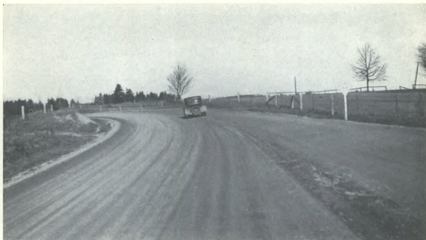
A. Illustrating smoothness of stabilized road surfaces: sodium chloride treated road at Schomberg, Ont.
