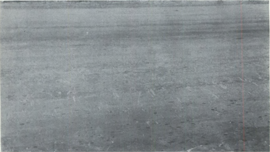
B. Illustrating hardness of sodium chloride treated road: tractor marks do not penetrate surface, Brechin, Ont.
