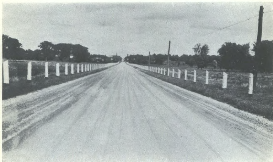
B. Illustrating smoothness of stabilized road surfaces: calcium chloride treated road near Wingham, Ont.
