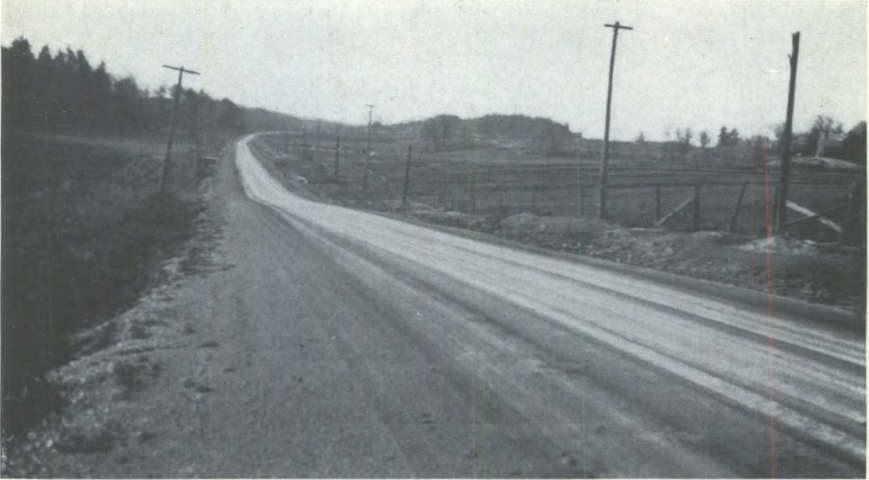
A. Whitish appearance of sodium chloride treated road in dry weather, east of Port Carling, Ont.
