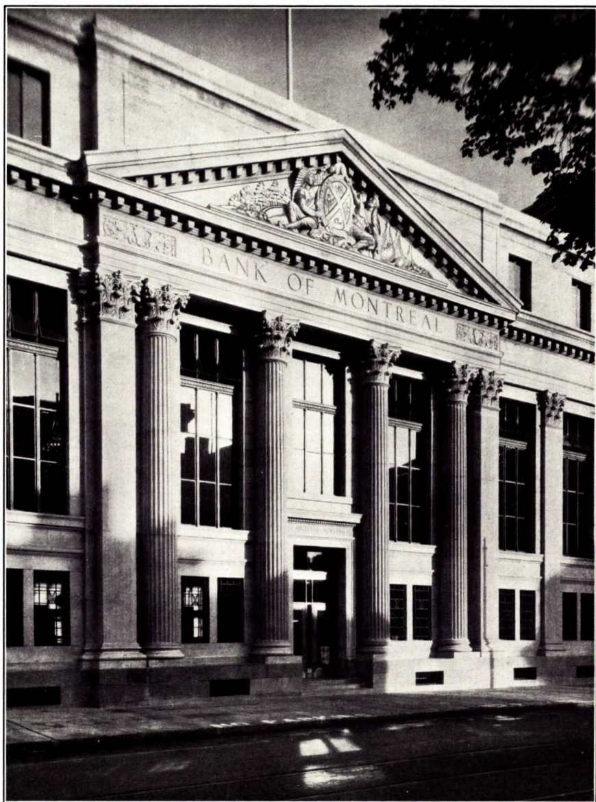
Photo. Pigott Construction Co., Hamilton.
