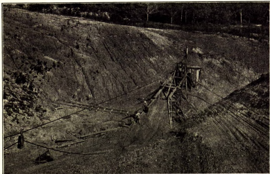
Drag scraper operating in thin clay bed.
