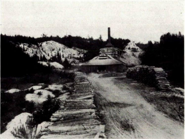
B. Lime plant of Purdy and Green, Ltd., Indiantown, Saint John, N.B. The wood in the foreground is fuel for the kilns.
