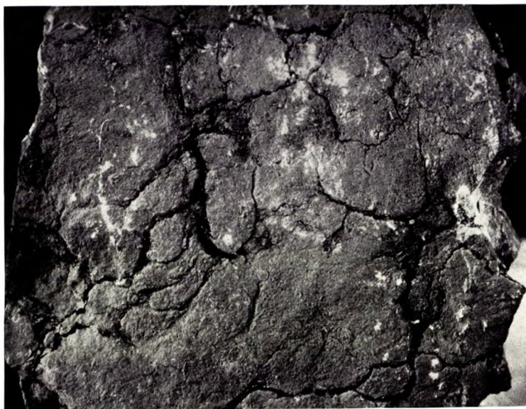
A. Cracked, weathered surface, typical of many Carboniferous calcium and high-calcium limestones.
