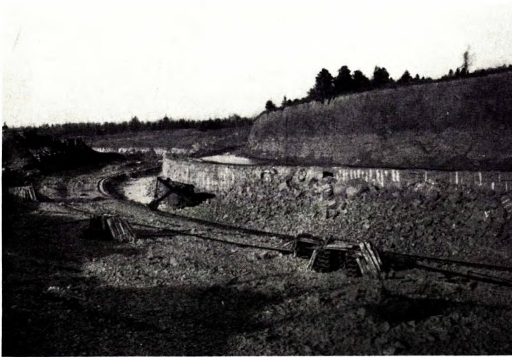
B. Quarry of Dominion Iron and Steel Corporation at Edwardsville, Cape Breton County, N.S., showing overburden removed from part of the limestone preparatory to quarrying the latter.
