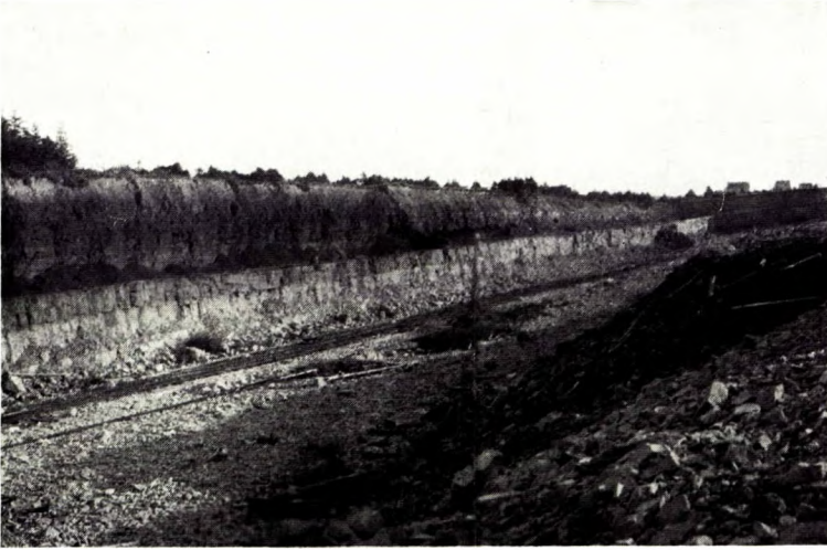
A. Quarry of Dominion Iron and Steel Corporation at Edwardsville, Cape Breton County, N.S. Southeast part of working-face showing dip of strata and depth of overburden.
