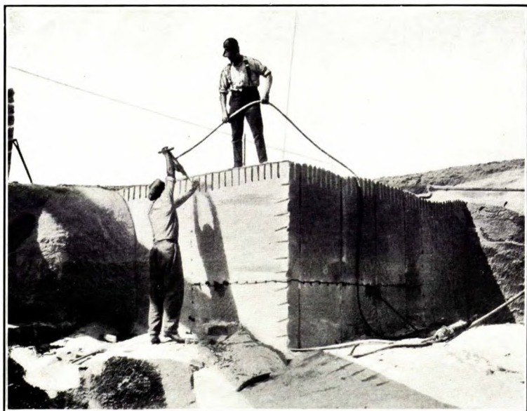
B. Method of splitting out a mill block at Queenston quarry, St. Davids, Ont.
