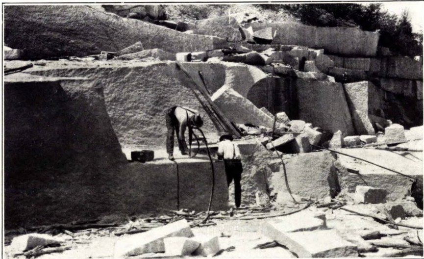
A. Breaking out curbstone, Quebec.
