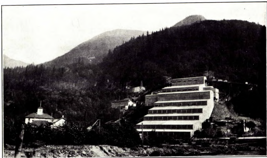
A. A concentrating mill at Britannia copper mine, British Columbia.
