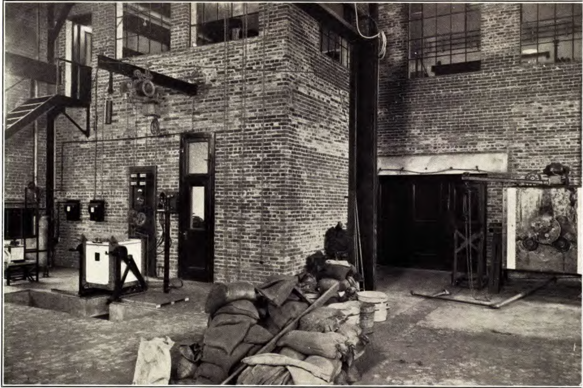
Part of the pyrometallurgical laboratory. On the left, Ajax high frequency induction furnaces with a capacity of 50 and 300 pounds respectively; on the extreme right, a rotary electric retort.
