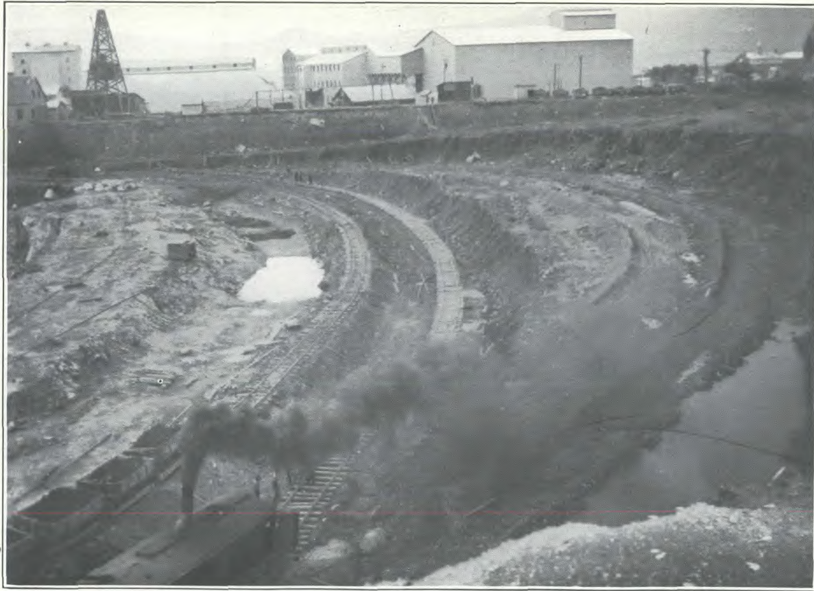
Steam shovel stripping overburden, King pit, Asbestos Corporation, Limited, Thetford Mines, Quebec.
