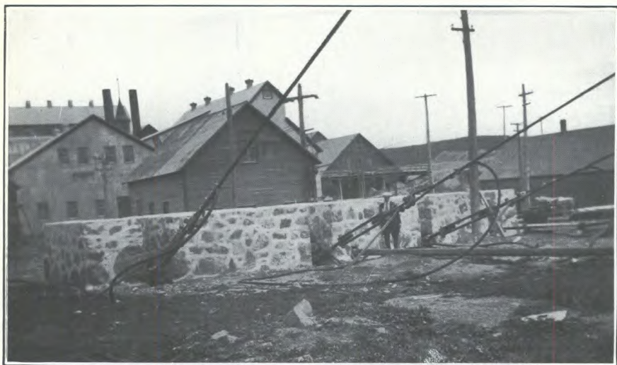
B. Deadmen for anchoring cables.
