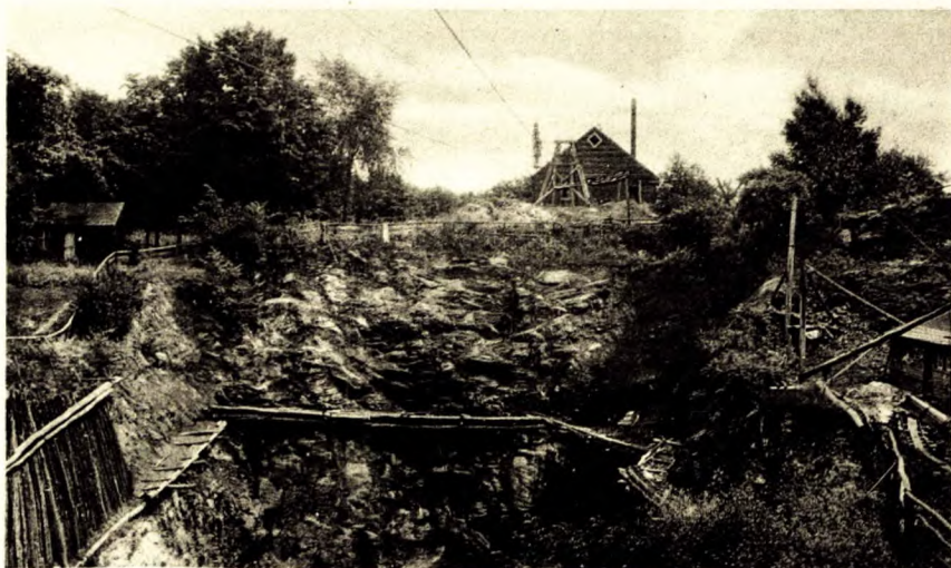
A. View of main pit, Lacey mine, concession VII, lot 11, Loughborough township, Ont. The strike of the mica leads is towards the hoist-house in the background, the principal vein (see Plate XV) passing approximately across the centre of the pit.
