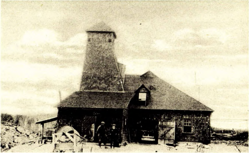
A. New shaft-house at Blackburn mine, rangé XI, lot 9, Templeton township, Que. The mica is rough-picked in the pit and dumped to the cobbing house in front of the hoist-tower, the clean, cobbed mica being shipped to the company's mica shop at Hull, Que.
