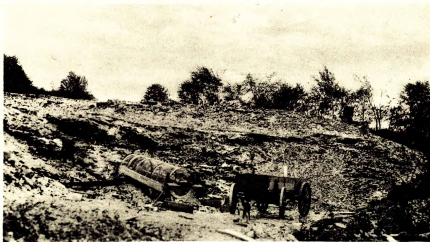
B. Portion of large dump, containing thousands of tons of shop-scrap mica, at Lacey mine, concession VII, lot 11, Loughborough township, Ont. The material of this dump, representing the accumulated waste from the trimming shop, is passed through the gasoline-driven screen, the oversize being shipped for grinding
