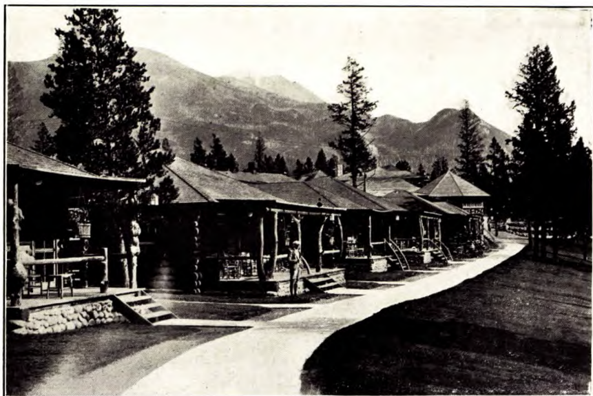
A. Walks at Jasper Lodge, Jasper, Alberta, surfaced with bituminous sand.
