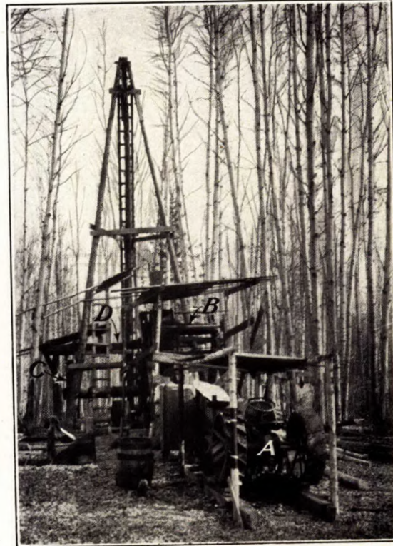
B. Equipment for core-drilling Alberta bituminous sand; A, Fordson tractor; B, draw-works; C, bull wheel; D, platform for connecting and disconnecting drill rods,
