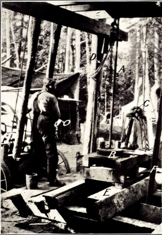
B. Rotary equipment for core-drilling Alberta bituminous sand: A, drill rod; B, rotary table; C, chain and sprocket for operating table; D, chain block; E, timber supports on which rotary table is moved aside; F, disconnected drill rods resting in cellar.
