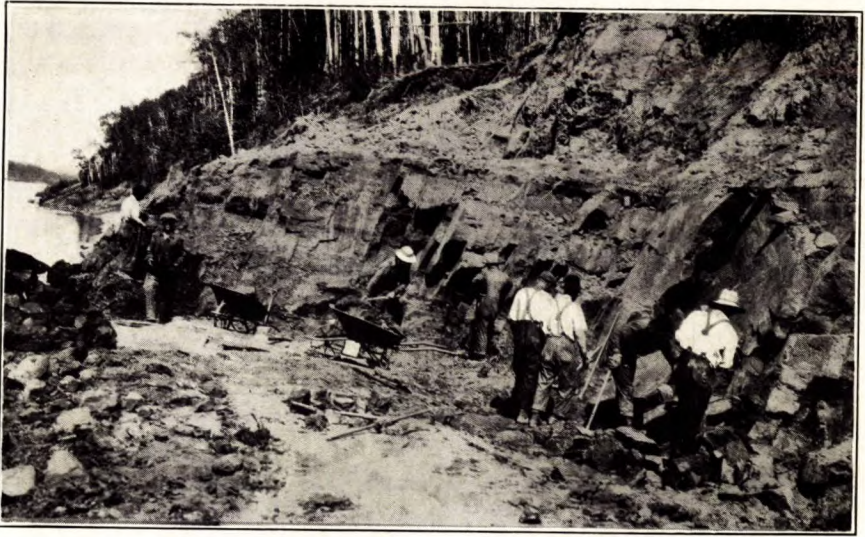
A. North end of bituminous sand quarry on Clearwater river, McMurray, Alberta, showing typical structure due to slipping.
