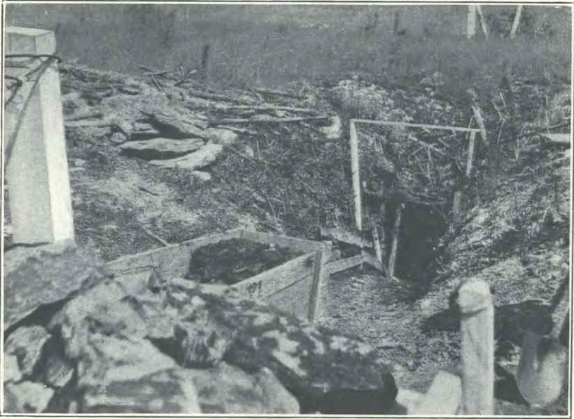
A. Mining oil shale, Rosevale, N.B. Tunnel entrance with freshly mined shale in the foreground.
