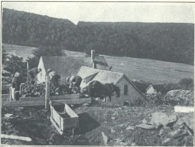
B. Mining oil shale, Rosevale, N.B. View from tunnel showing shale and loading platform.
