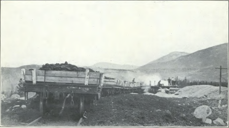
A. First commercial shipment of Alberta bituminous sand for road-surfacing purposes arriving at Jasper.
