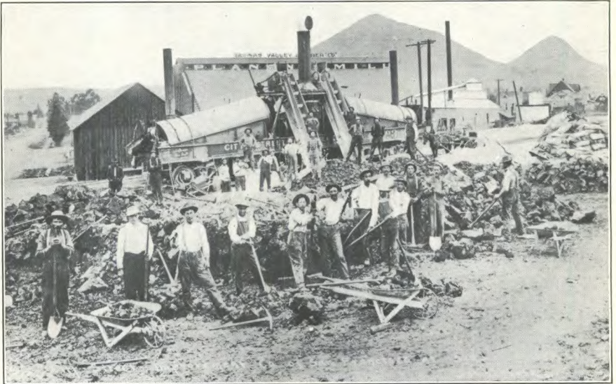
B. Portable, externally heated mixing plant (railroad type), California.
