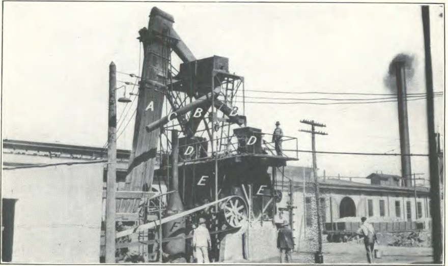
A. Two-drum, internally heated mixing plant; Uvalde Rock Asphalt Company, San Antonio, Texas. A, elevator; B-B, discharge chutes from elevator; C, dust catcher; D-D, feed hoppers; E-E, mixing-drums (8 feet diameter and 6 feet long); F, steam boiler.
