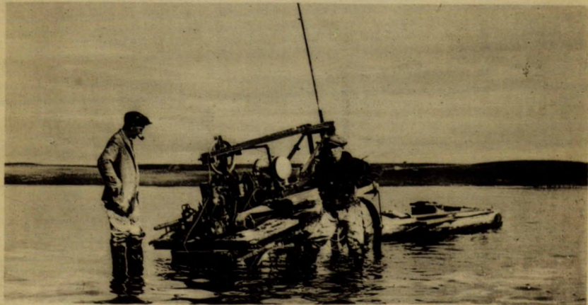
B. Drill sunk in mud hole, Snakehole lake, Sask.
