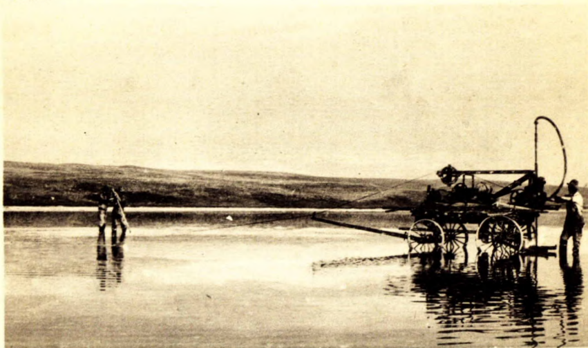
A. Method of moving drill by its own power, Vincent lake, Sask.
