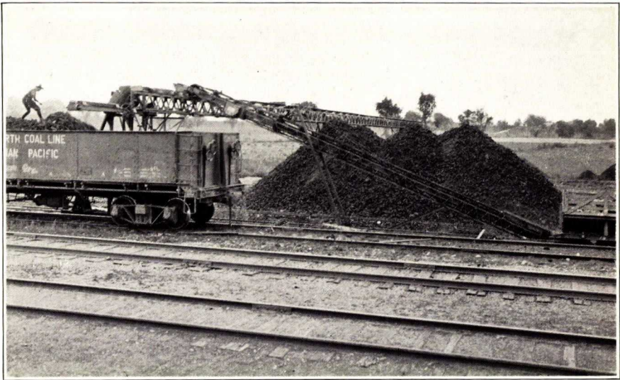
View of loading and storage conveyer showing elevator
