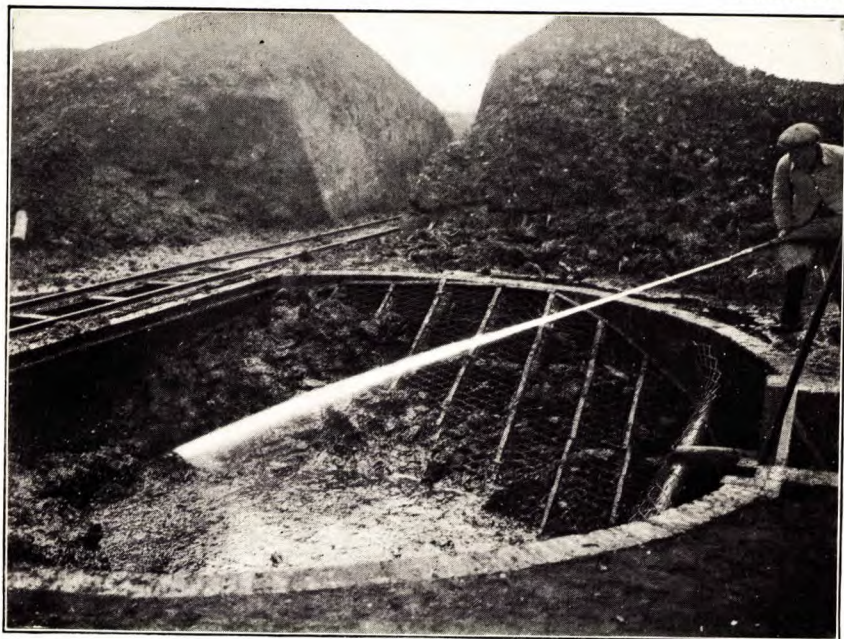
Masonry tank, with expanded metal bottom, used in Migeon process.
