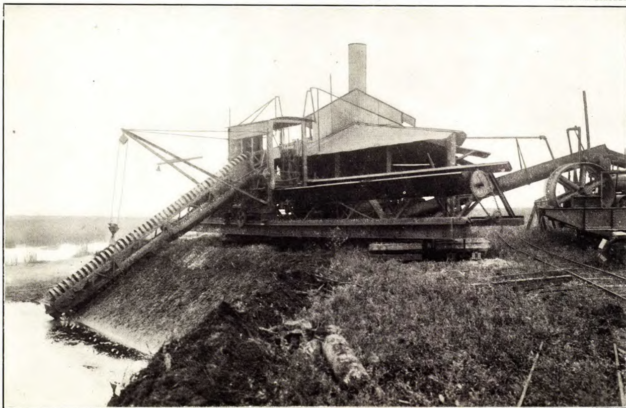
Peat Committee's Plant No. 1—excavator
