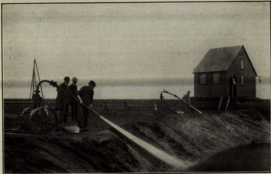
Hydraulic excavation of peat on Lundergaard bog, Denmark
