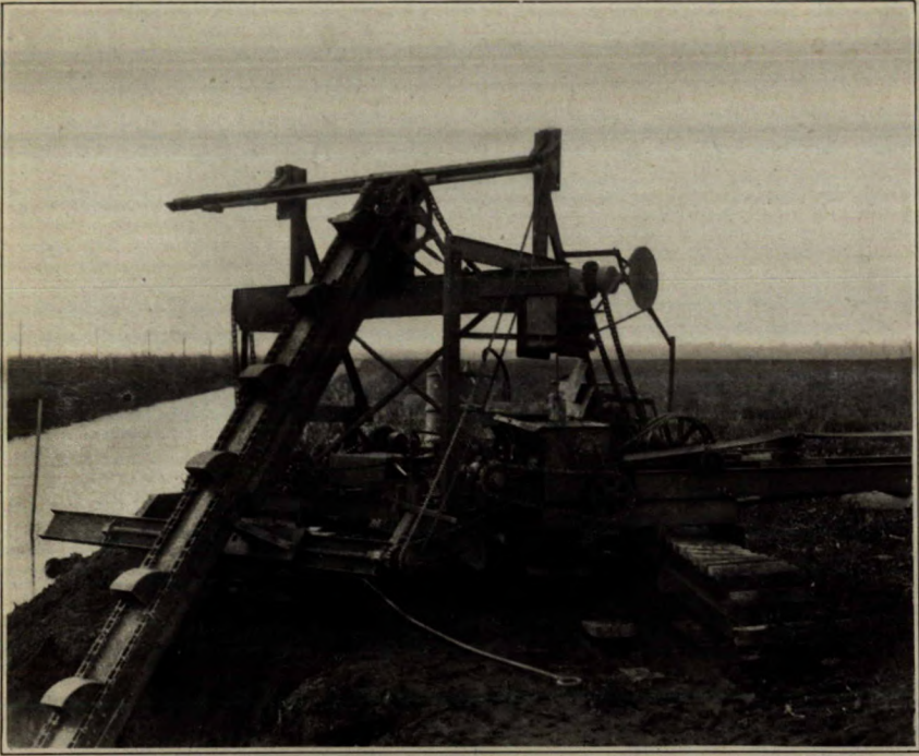
Plant No. 3—excavator, second design
