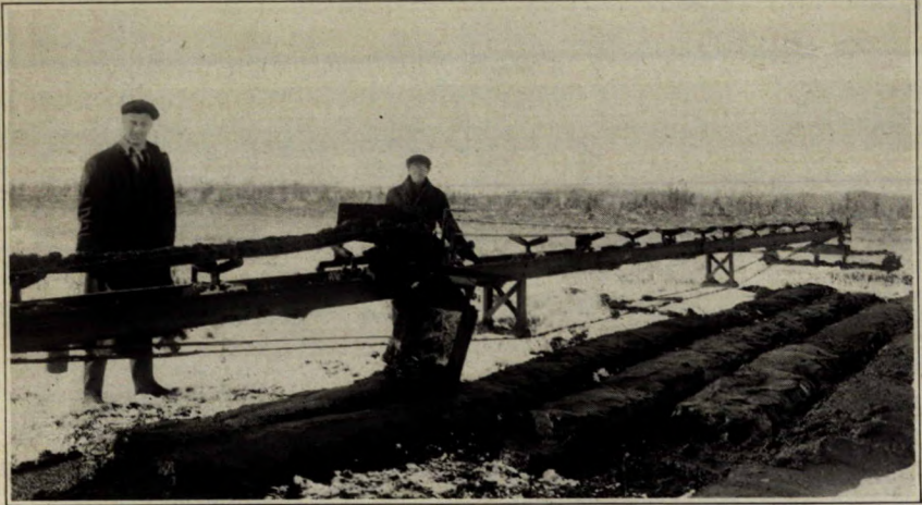
Plant No. 3—spreading system
