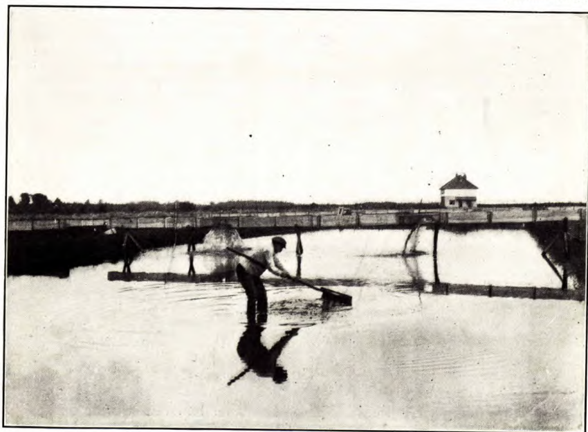
Stationary conduit leading to drying-area, used in Migeon process.
