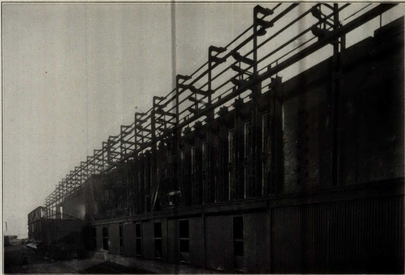
View along coke side of Wilputte ovens, showing the coke-quenching car, coke guide, door machine, and clay carrier.
