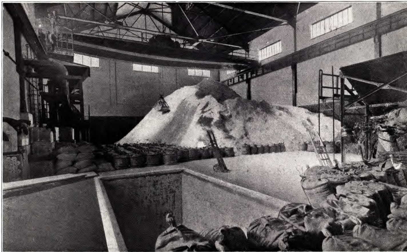
Sulphate storage room, Colorado Fuel and Iron Company, Pueblo, Col.
