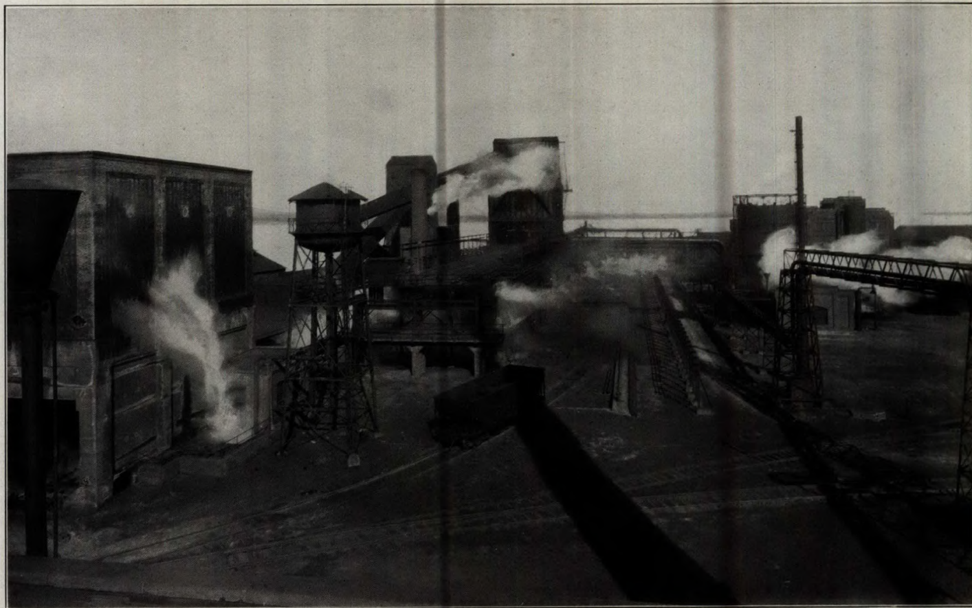
Bird's-eye view of Wilputte by-product coke oven plant, Hamilton. Quenching hood and water tower in left foreground; by-product building in right background.
