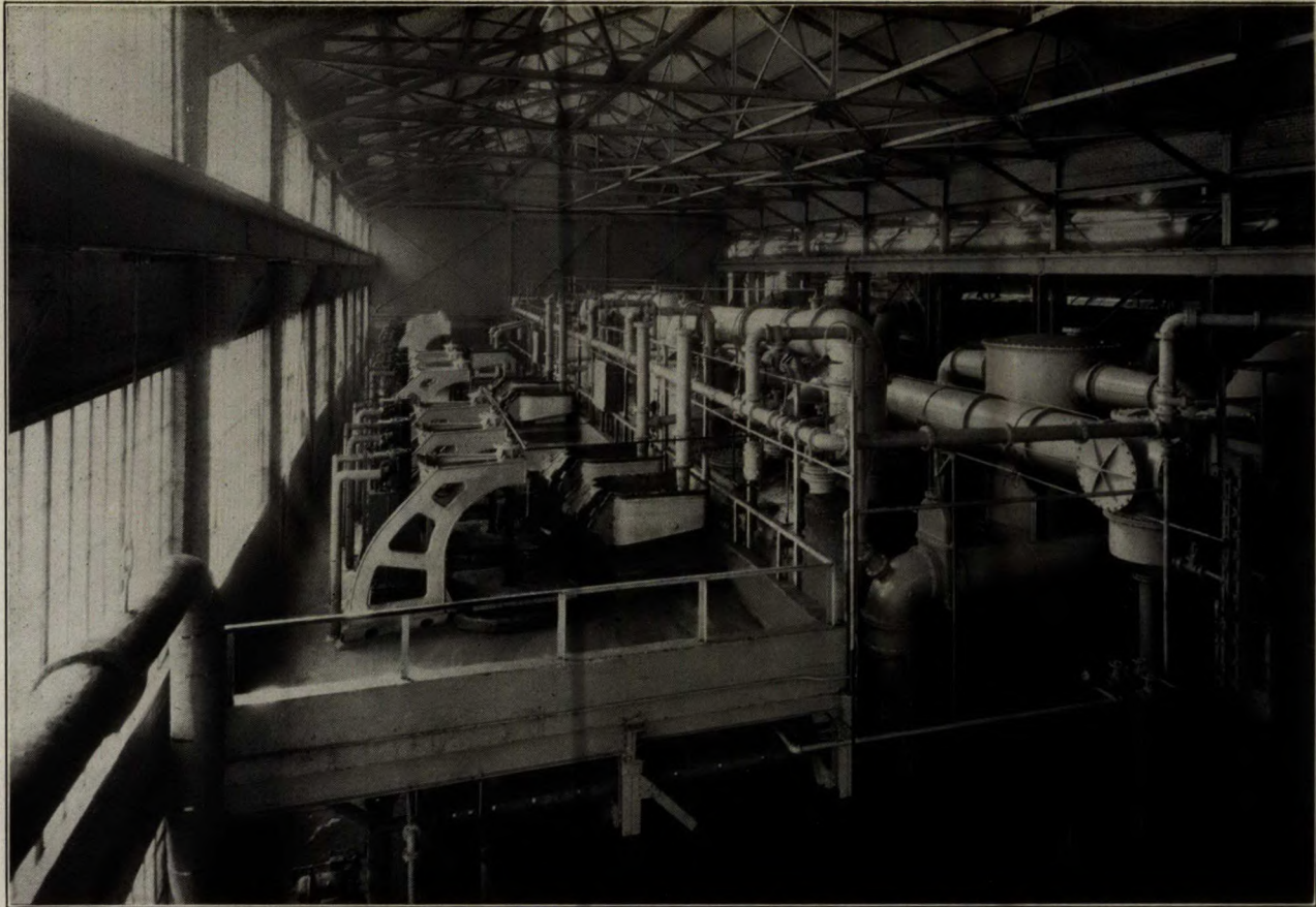
Typical installation, ammonium sulphate plant. Note centrifuges, saturators, piping, etc.
