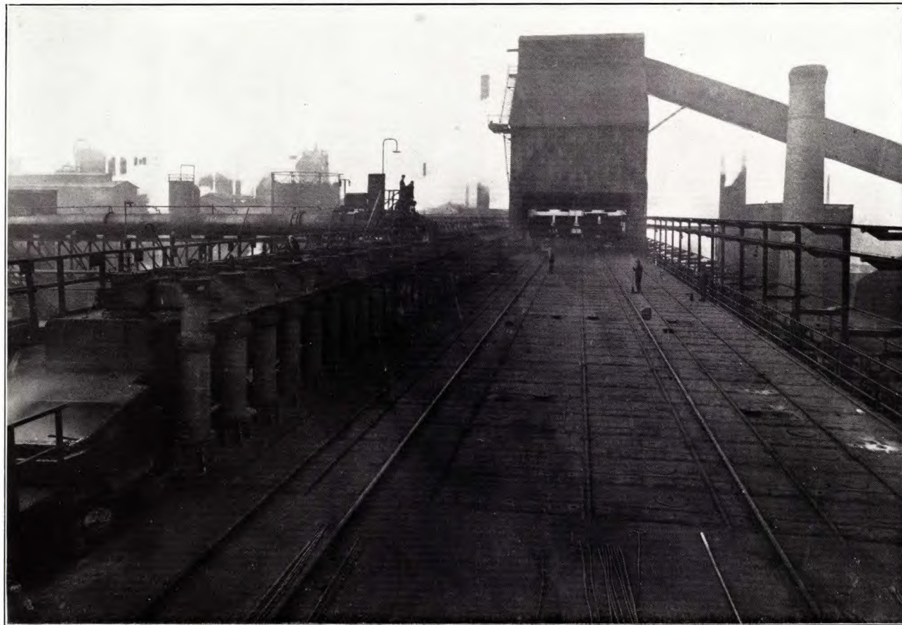
Top of Wilputte ovens with coal bin in centre background under which stands the four-hopper larry car.
