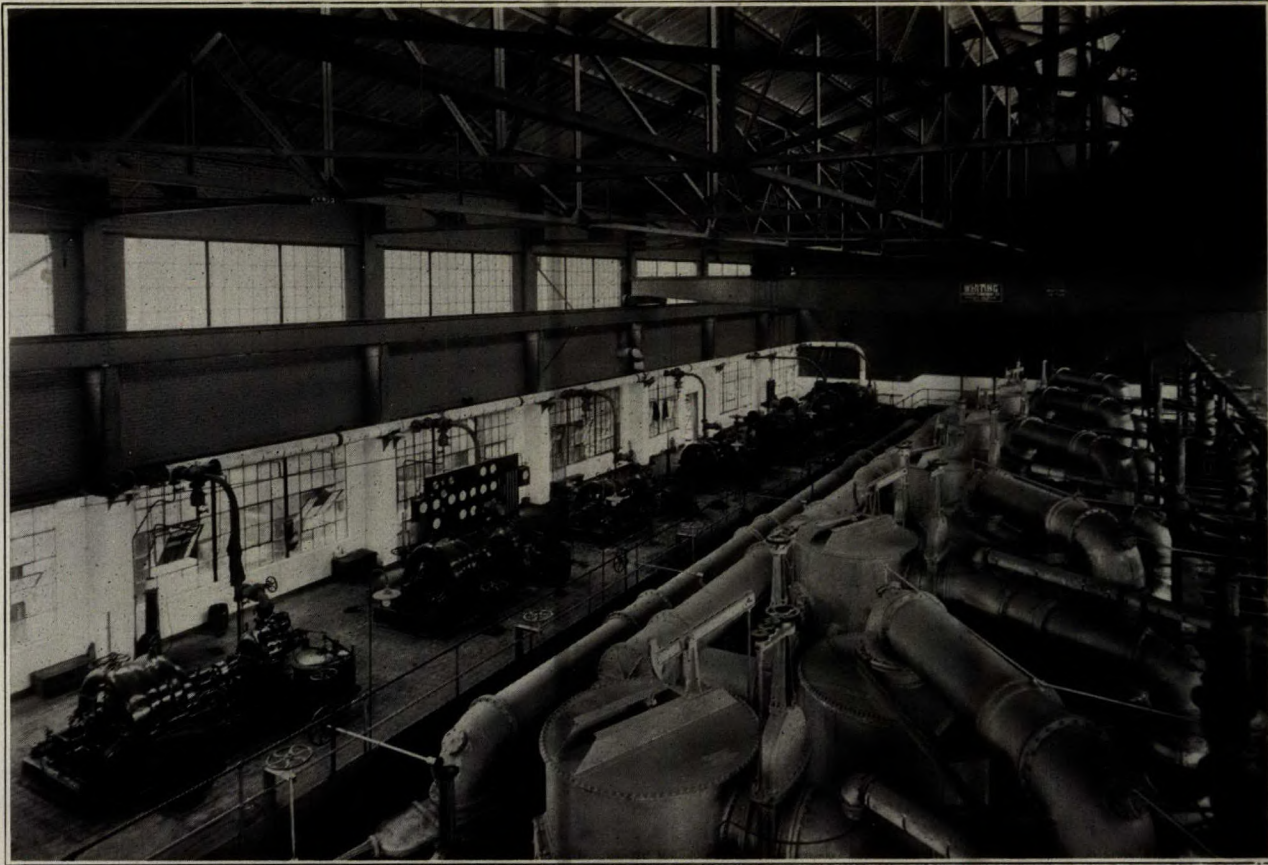
Interior of by-product building, Cambria plant, Bethlehem Steel Company. Note exhauster, saturaters, etc.
