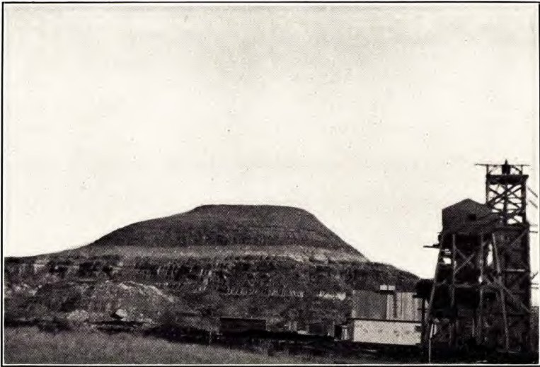
Typical small butte in Red Deer valley, near Drumheller, Alberta. A bed of bentonite, 3 feet thick, occurs just below the light-coloured band half way up the slope. Thin bentonite beds occur similarly in many of the buttes up and down the valley and in the cliffs forming its sides.
