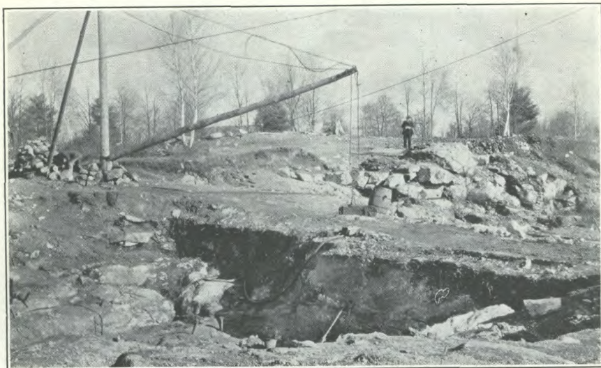
Chisholm mine, Sheffield township, Ont. No. 1 pit, looking east. Bottom of this pit is solid iron sulphides carrying molybdenite.
