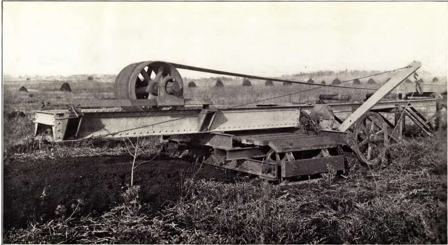
One of the caterpillar elements, and take up pulley at extreme outboard end of the conveyer
