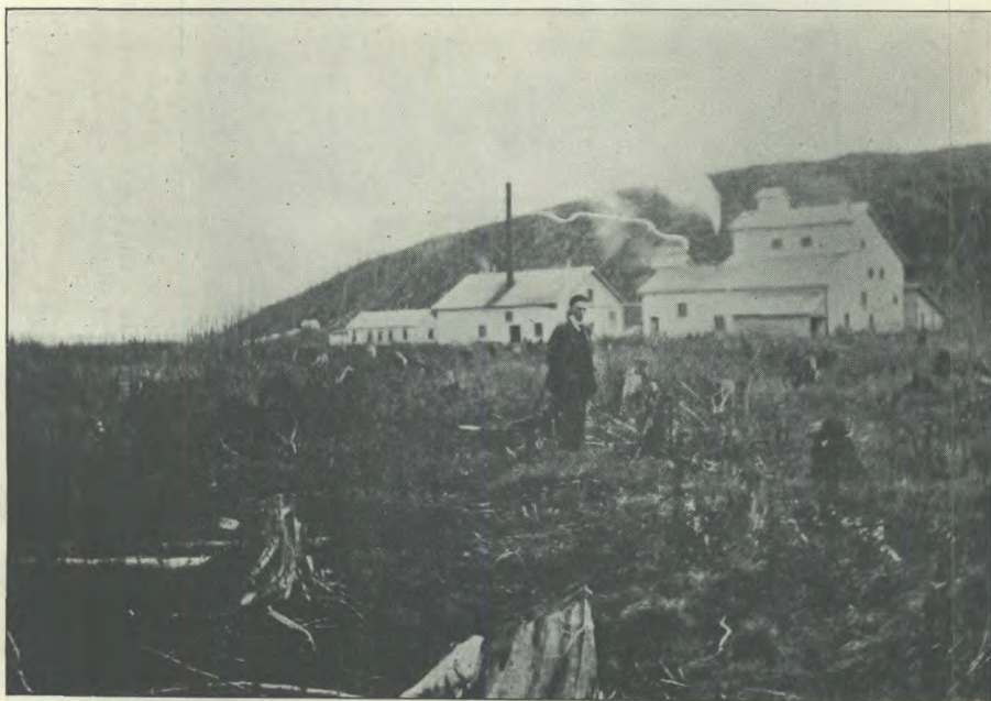
General view of property of Premier Langmuir Mines Ltd., township of Langmuir, northern Ontario, showing mill and part of outcrop of vein.
