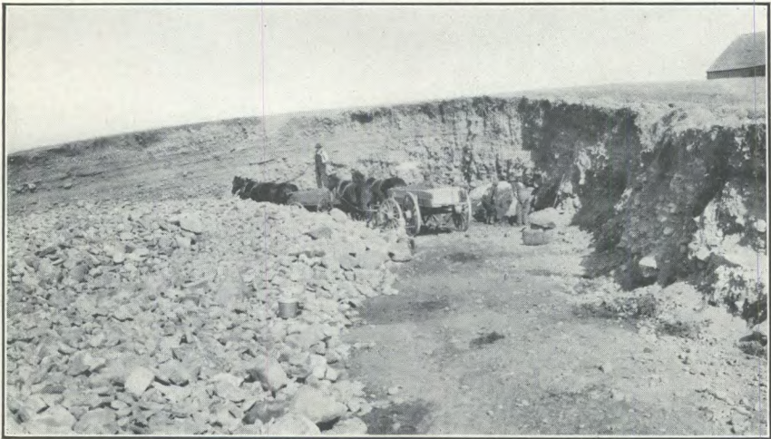
Gravel pit, showing stratification and bed-rock floor.
