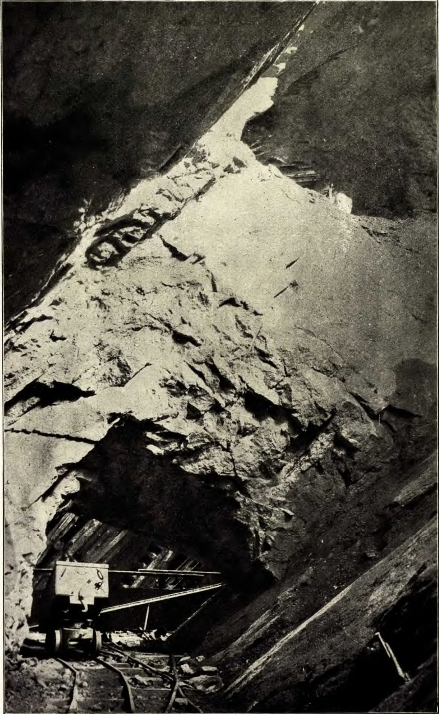
100-foot level at mine of Globe Graphite Mining and Refining Company, concession VI, lot 21, township of North Elmsley, Ont. The pillar indicates the thickness of the ore-body in the east workings.
