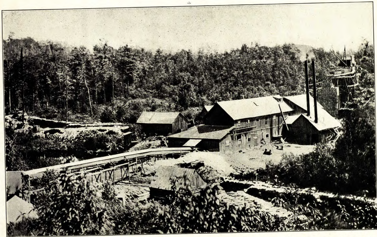
Mill of the Buckingham Graphite Company (North American mine), township of Buckingham, Que. The photograph was taken some years ago, and the buildings are now in a dilapidated condition. The strike of the ore-body is indicated by the tramway, and the main drift enters the mill to the left of the kiln.
