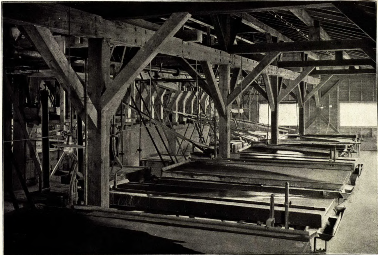
Section of mill, showing Krupp-Ferraris tables, slime tables and hydraulic classifiers, New Quebec Graphite Company, Buckingham, Que.
