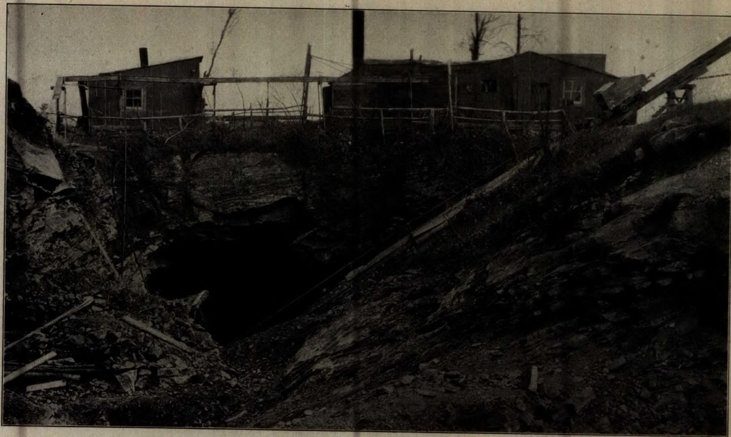
Open cut above workings of Globe Graphite Mining and Refining Company, concession VI, lot 21, township of North Elmsley, Ont. The banding in the limestone is well shown, and a well defined fold is exhibited in the cap rock above the shaft. Graphite bodies tend to occur at the crests of such folds.
