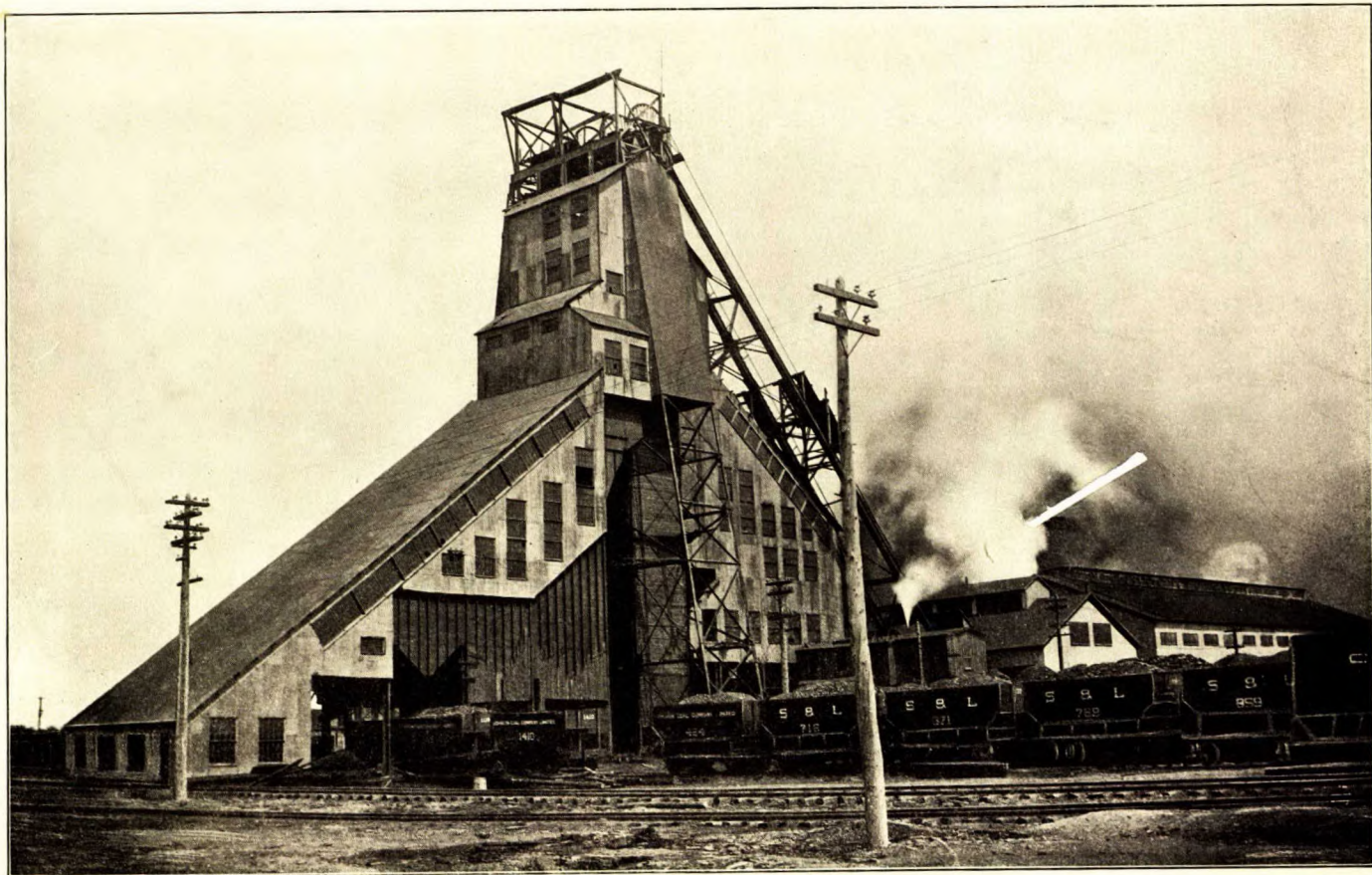
Nos. 2 and 9 Collieries of the Dominion Coal Company: two coal seams are worked at this mine to contiguous shafts.
