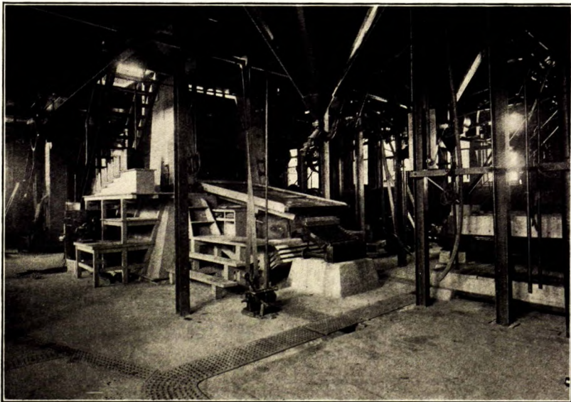
Ore dressing laboratory: view on first floor, Callow tanks, stamp battery cyanide zinc boxes.
