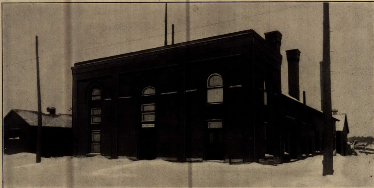
Fuel testing station and ore dressing and metallurgical laboratory.
