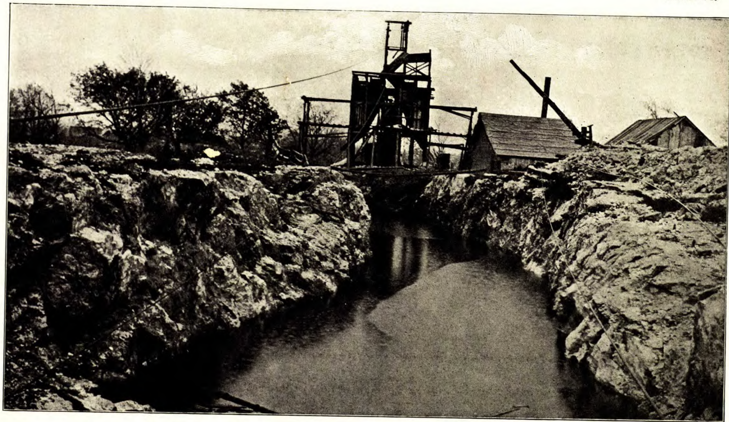
Card quarry, Portland township, Ont.: showing open-cut and cable hoist.
