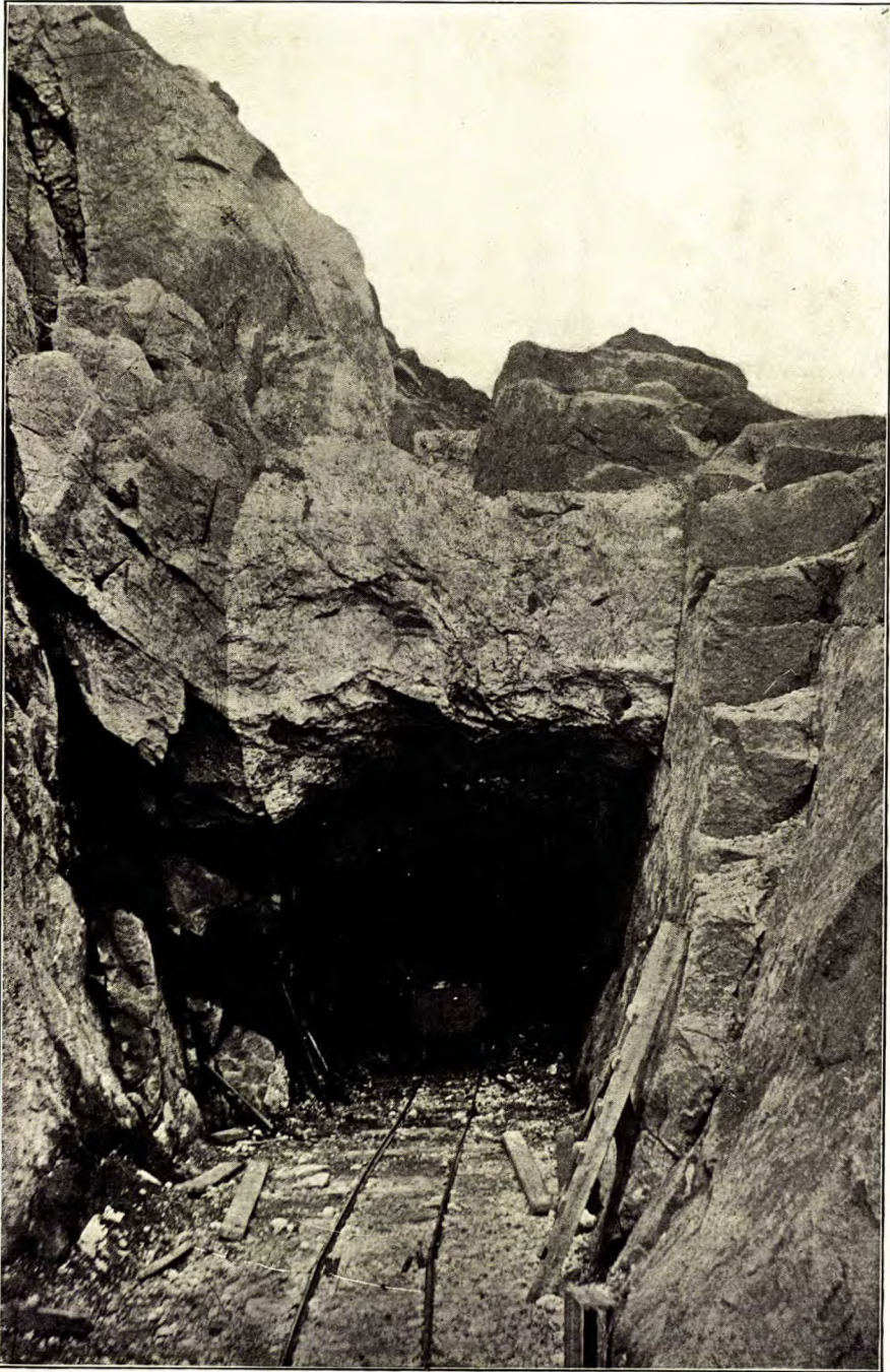
Method of working feldspar dike, Mosken, Lofoten islands, Norway.
