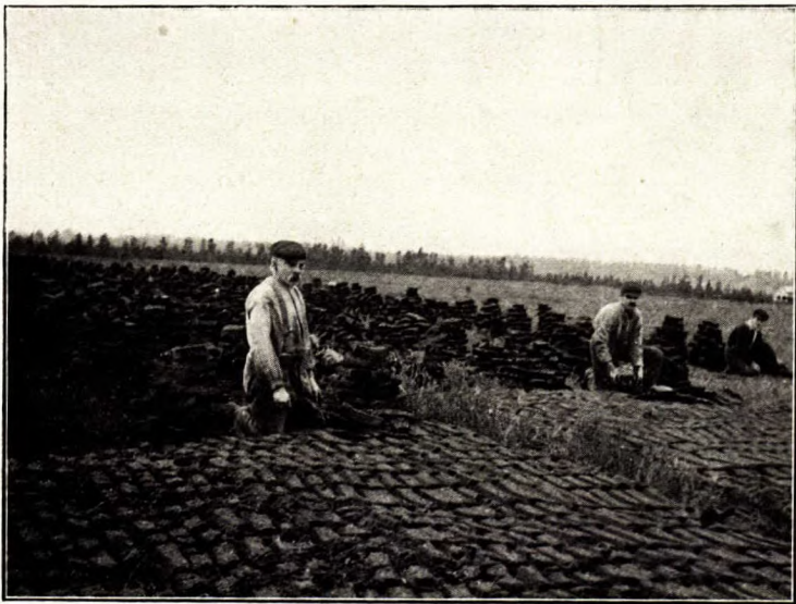
Piling peat into hives (cubes). This peat has not been turned. Alfred, Ontario.
