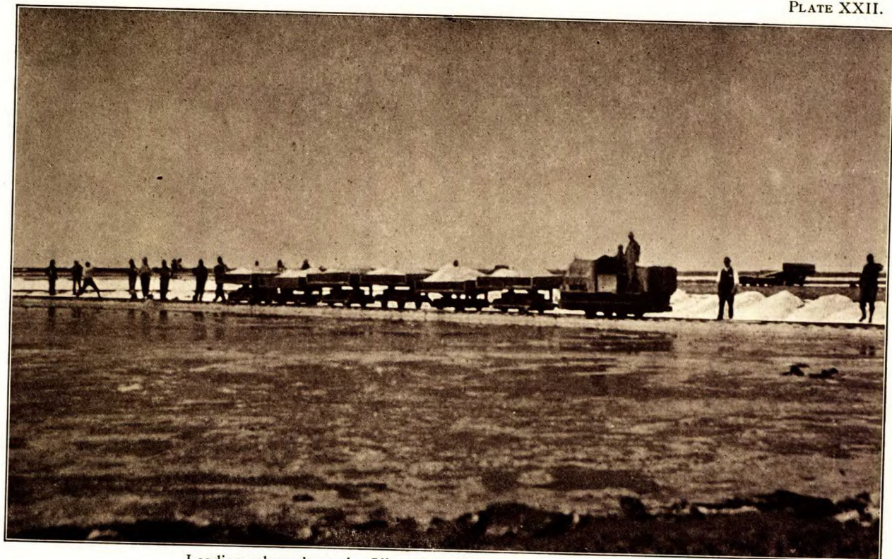
Loading solar salt at the Oliver Salt Co.'s plant, Mt. Eden, California.
