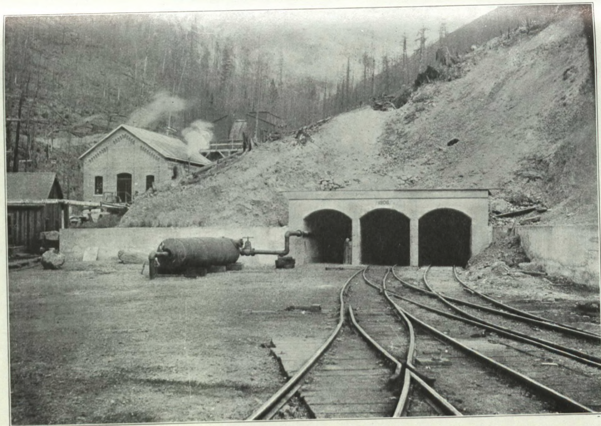
Mines Hosmer: tunnel principal, Hosmer, C. B.
