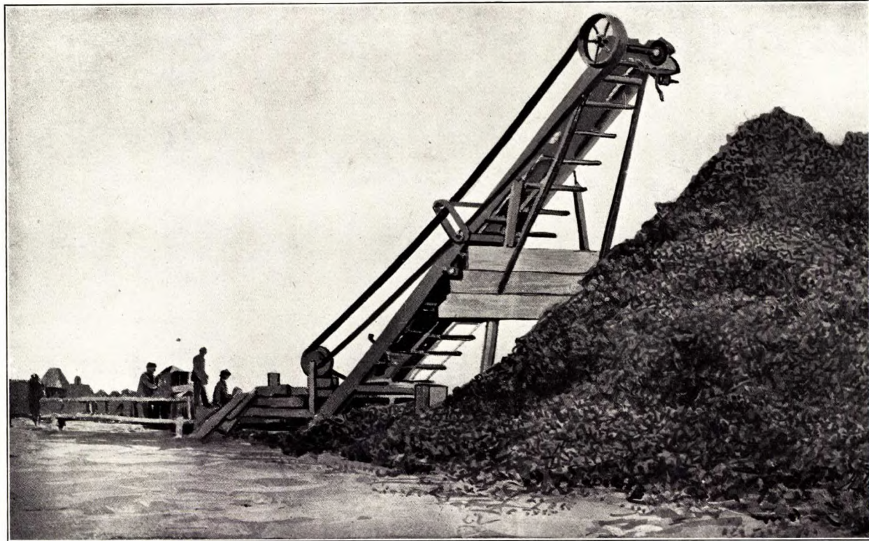
Peat elevator in operation.
