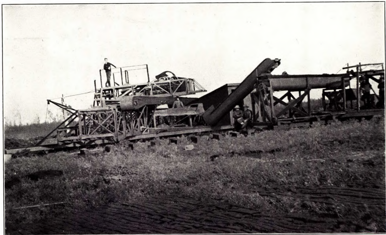
Loading hopper and buckets: Anrep automatic peat excavator.
