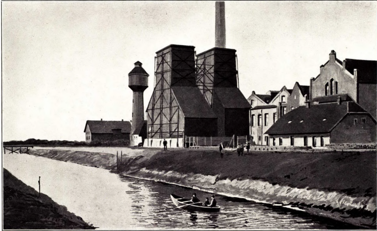
Completed portion of canal in front of power house.
