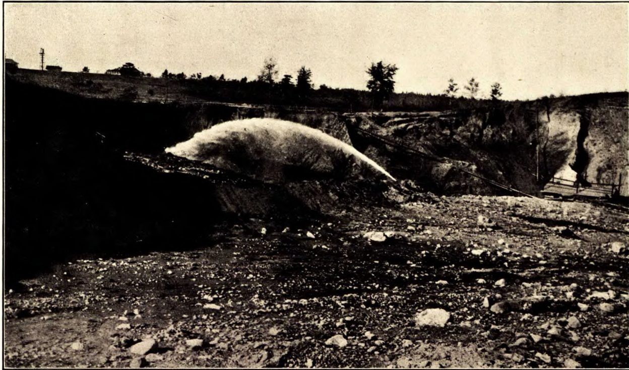
Rowe mine, Minnesota. General view illustrating hydraulic removal of overburden and showing water supply pipe, discharge pipe, and hydraulic gun.
