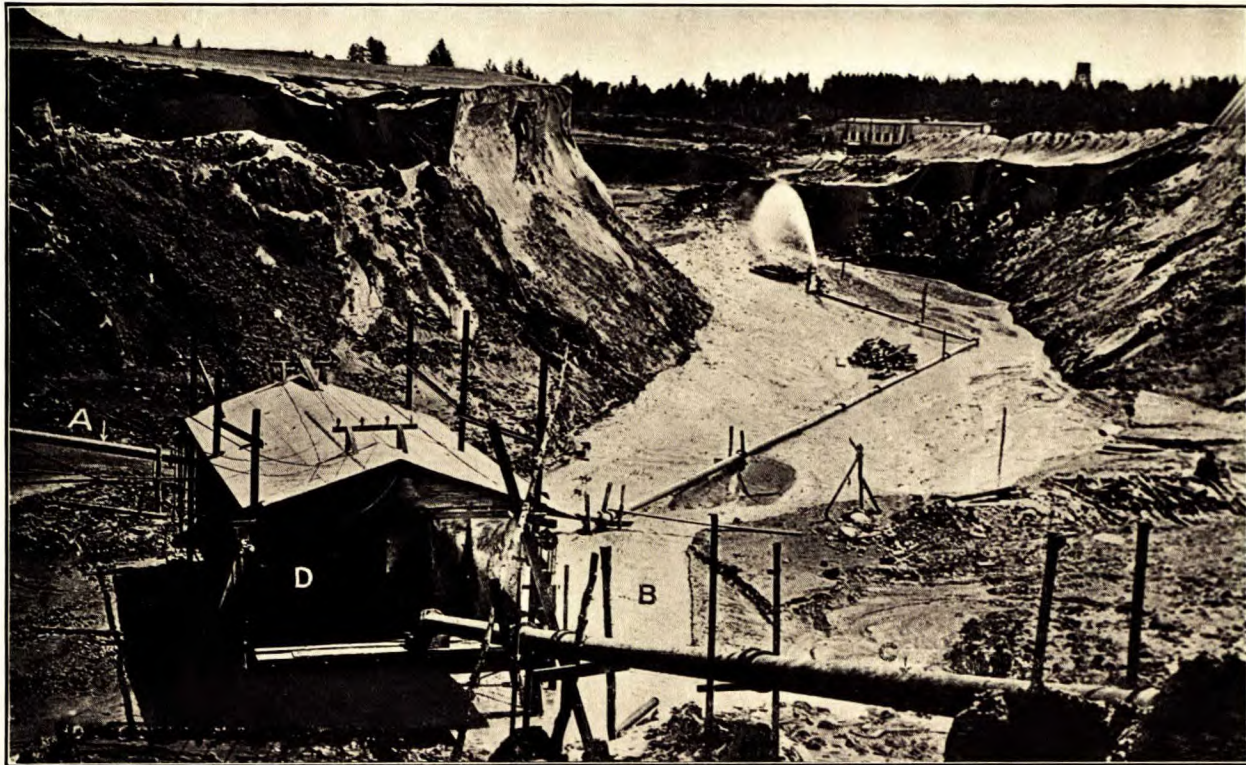
Rowe mine, Minnesota. Illustration of general arrangement of plant for removal of overburden by hydraulic stripping. (A) Water supply pipe to hydraulic gun. (B) Sump. (C) Discharge pipe leading from centrifugal pump. (D) Housed platform suspended from columns driven to bed-rock and carrying centrifugal pump and motor.
