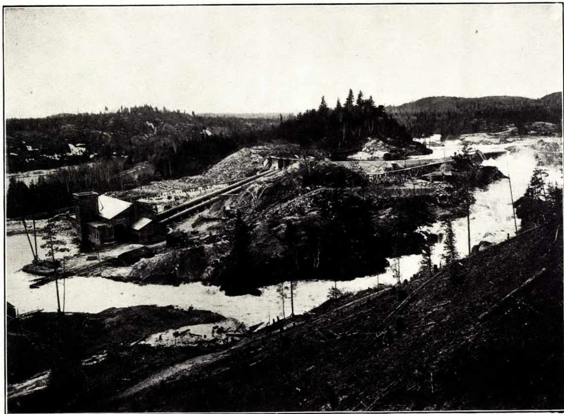
Usine génératrice de High Falls, Spanish River, "Canadian Copper Co."
