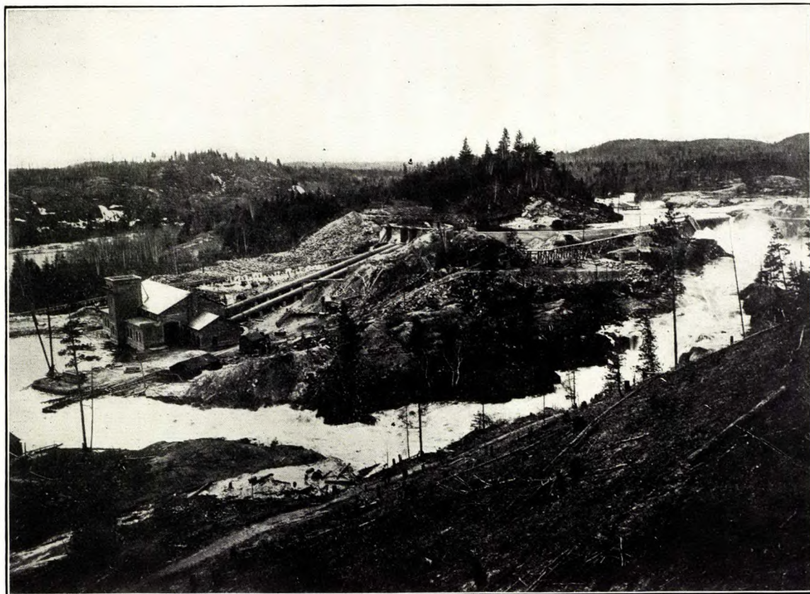
Power plant, High Falls, Spanish river, Canadian Copper Co.
