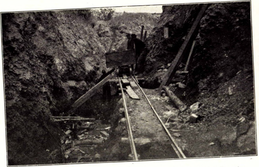
Dumping ore from open cut into chute, through upraise from lower level, Lone Star mine.
