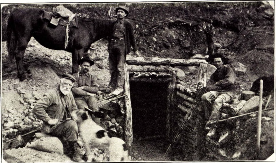
Tunnel entry, the Olive mineral claim.
