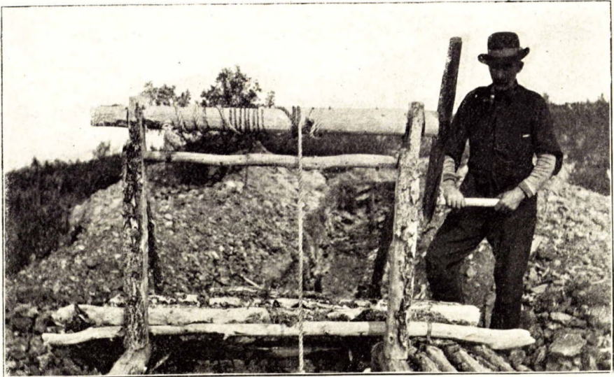
Shaft and trench on Jack Pot mineral claim, Box Car group. Mr. Sam. Thurbur at the windlass.
