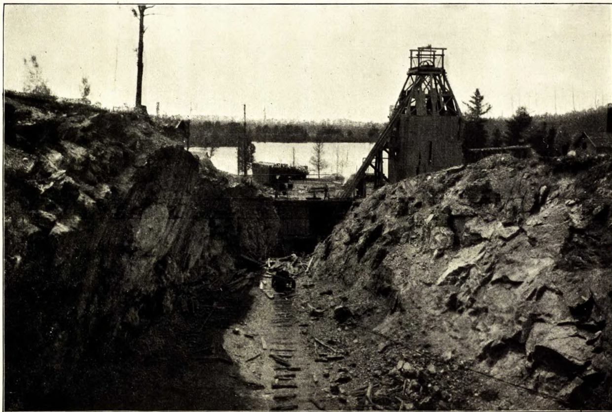
Open cut of No. 4 mine at Bessemer.
