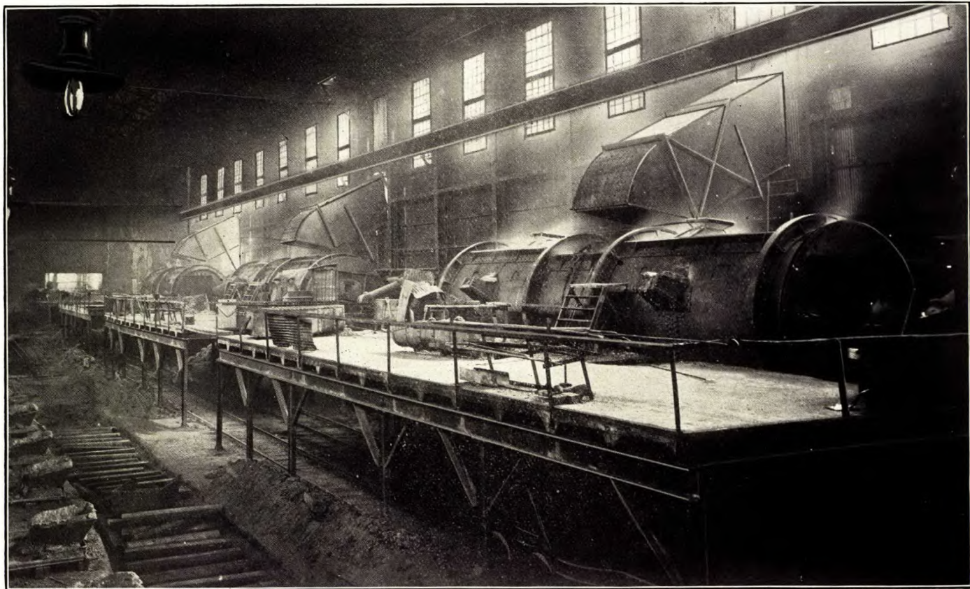
Basic converters, Canadian Copper Co. smelter, Copper Cliff.
