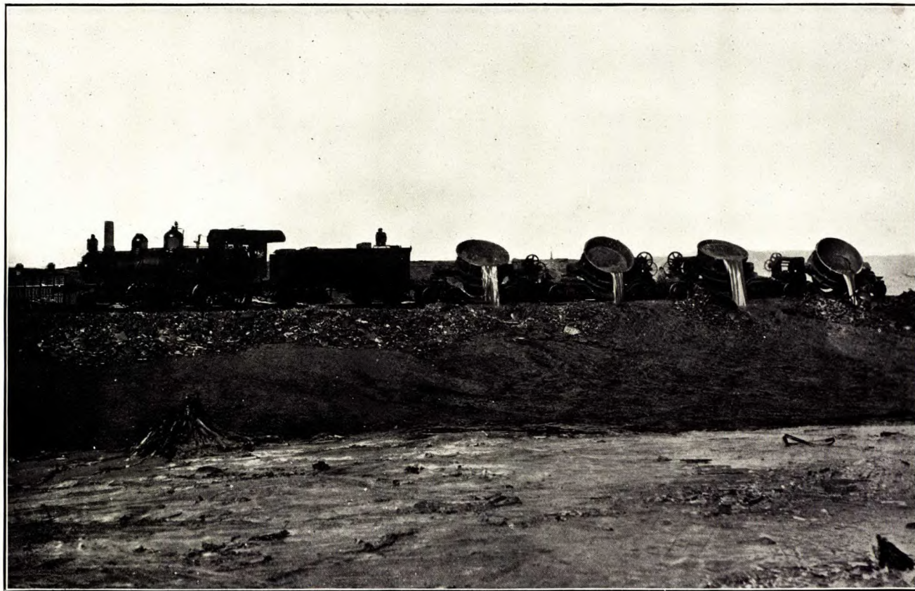
Pouring slag: Canadian Copper Co. smelter, Copper Cliff.
