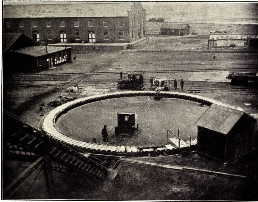
Slag cooling machine: Canadian Copper Co. smelter, Copper Cliff.
