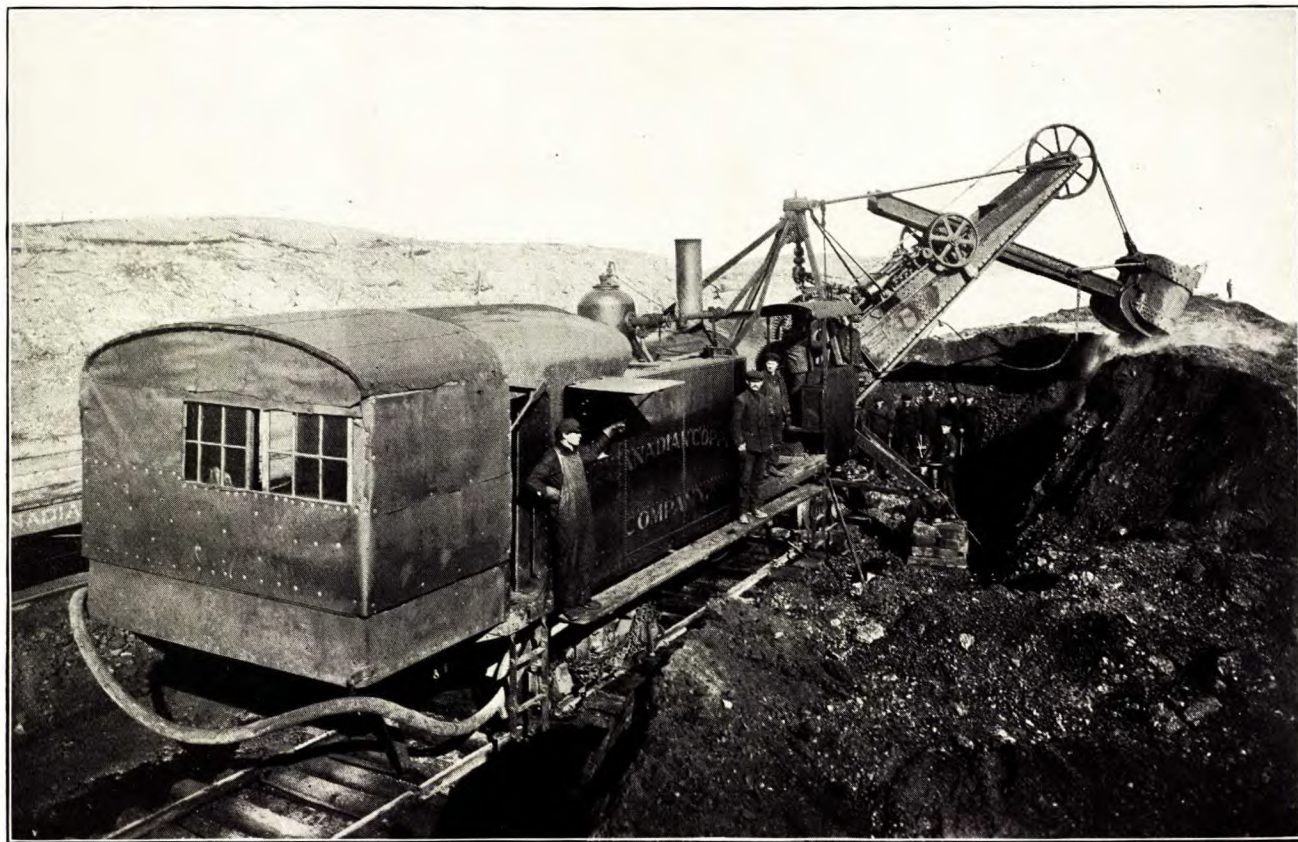
Canadian Copper Co. steam shovel at roast yard, Copper Cliff.
