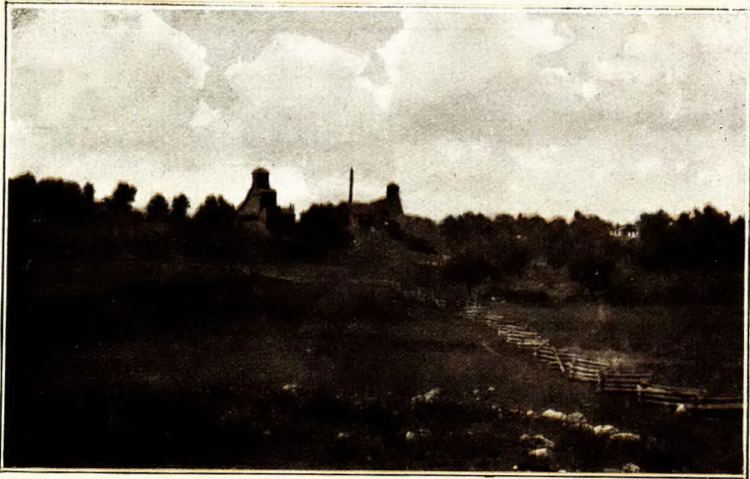
A. Head frames at the Sulphide mine, Nichols Chemical Company.
