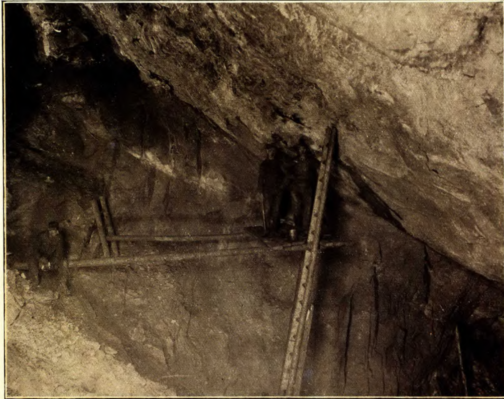
Eustis mine. Mining ore, main stope near 21st level.
