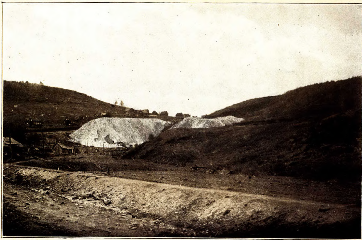
Eustis mine. Showing dumps and tram line to mill.
