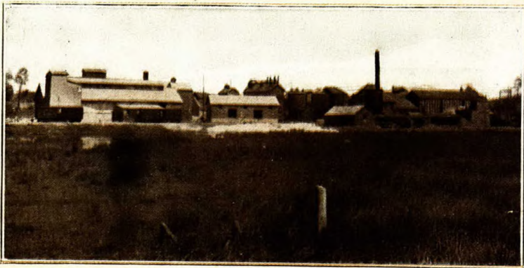
C. General view of the acid works, Sulphide, Ontario. Views at Sulphide, Ontario.
