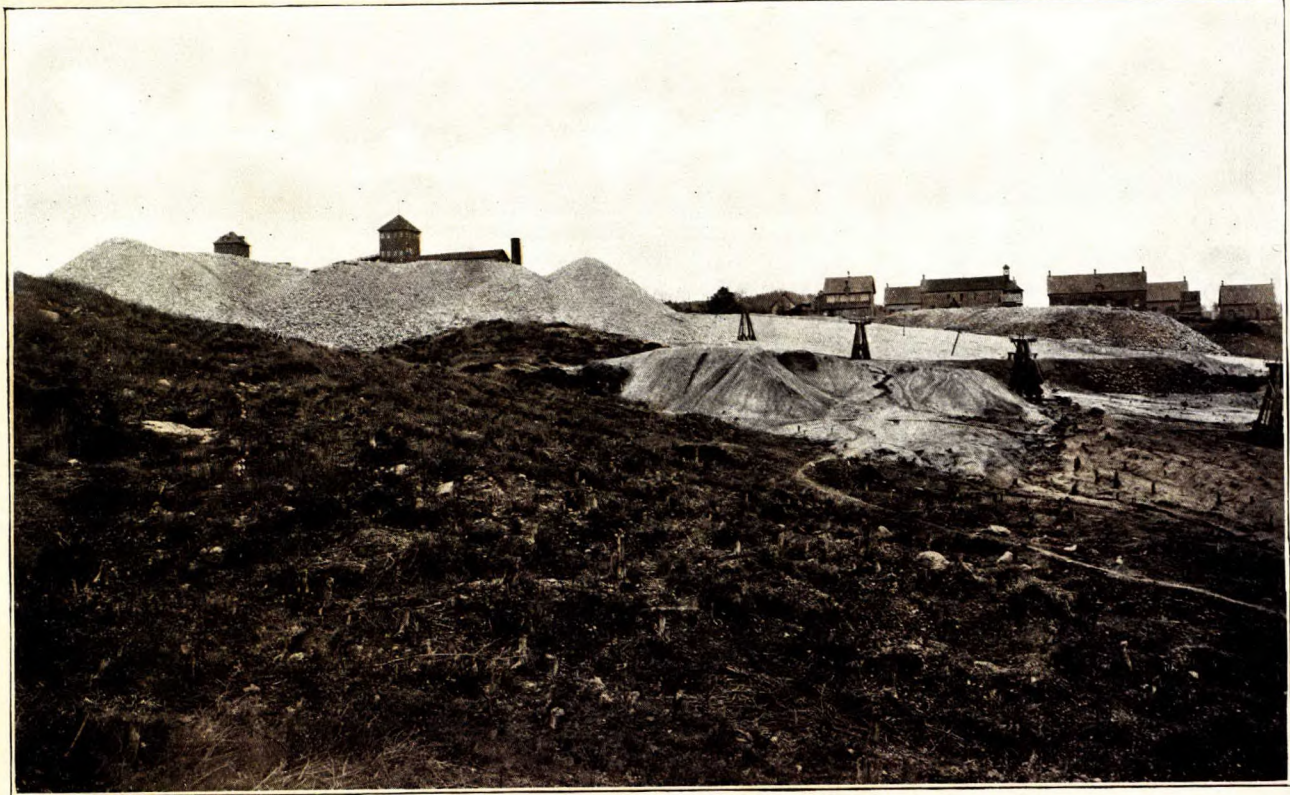
Albert mine. Shaft house, dumps, and tailings.
