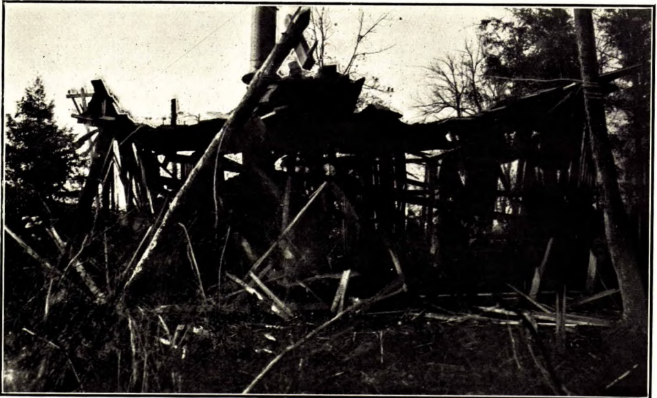
Explosion of one ton of 60 per cent dynamite in mixing house, showing damage to boiler house.
