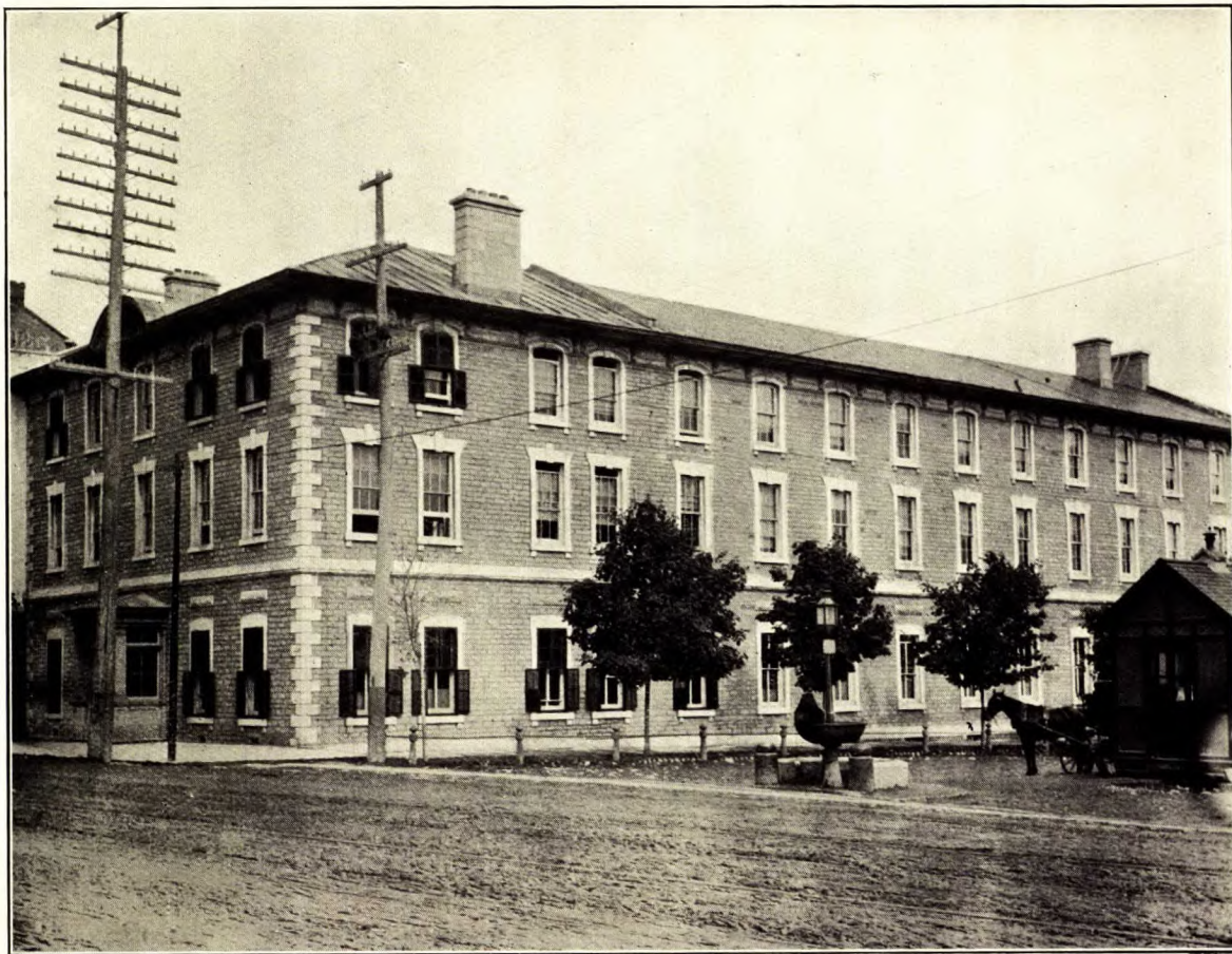
New headquarters of the Mines Branch of the Department of Mines, corner of Sussex and George Streets, Ottawa.
