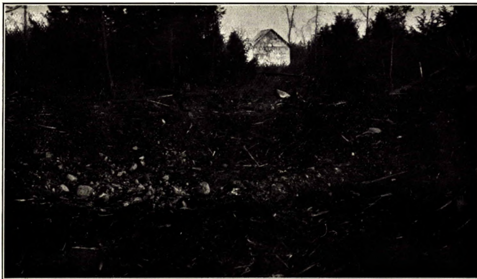
Site of mixing house with expense magazine in the distance : where about 150 cases of dynamite were stored. About one ton of 60 per cent dynamite exploded in the mixing house.
