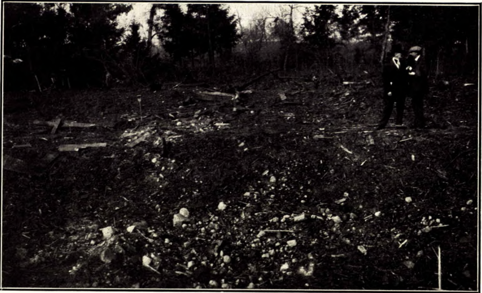
Explosion in mixing house, showing damage to boiler house.
