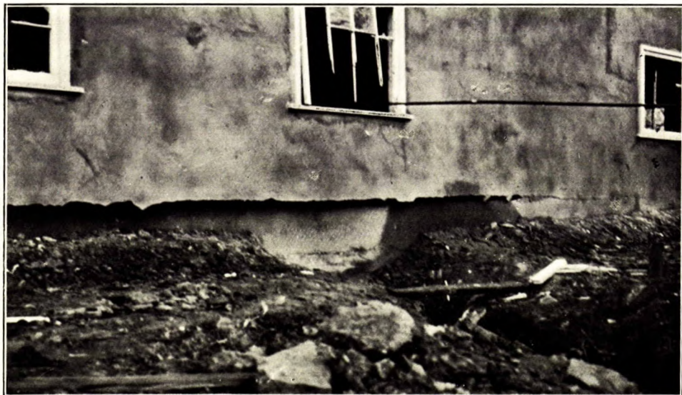
Explosion of one ton of 60 per cent dynamite. This house is at the acid plant 600 yards from the mixing house. Building constructed of reinforced concrete. See effect of suction.
