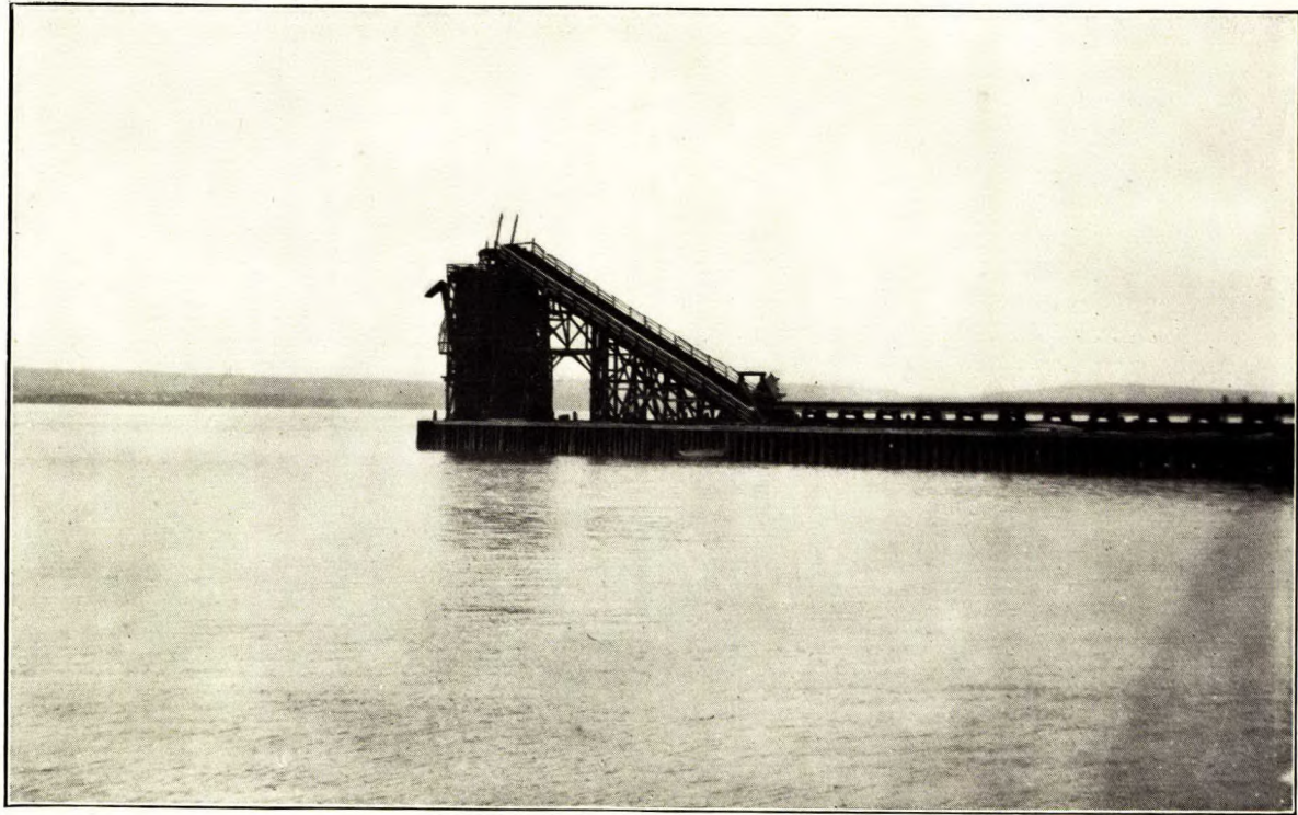
Loading pier, showing conveyer, Port Wade, N. S.
